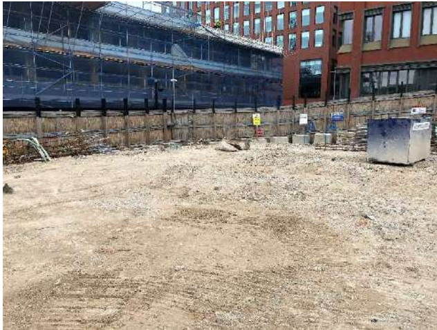
Photo 5 – Majority of northeast corner of site awaiting piling (due to start 19 th October)
