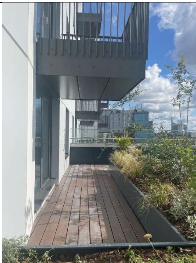
Photo 7 – Completed planters on Level 7.
