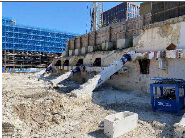
Photo 9 – Retaining wall on the eastern site boundary. Piles installed in between current steel supports.
