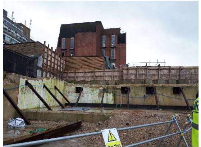
Photo 6 – Retaining wall in north east of the site
