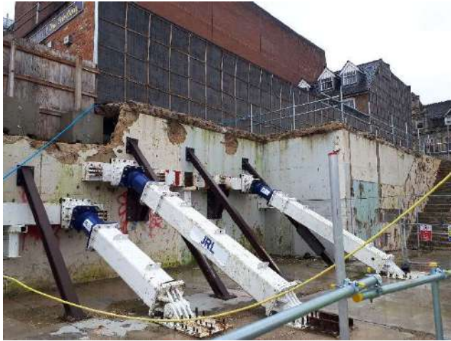
Photo 5 – Retaining wall along eastern boundary
