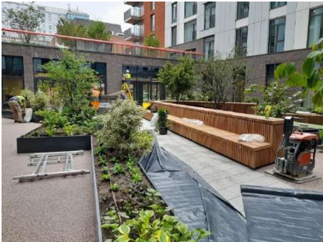
Photo 6 – View of soft landscaping in Block E courtyard south.
