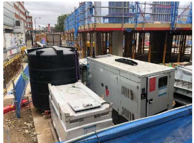
Photo 6 – Block E construction plant appropriately stored on concrete hardstanding.
