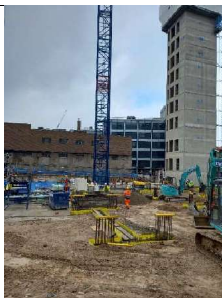
Photo 2 – View facing northwest showing ongoing construction of Block E.
