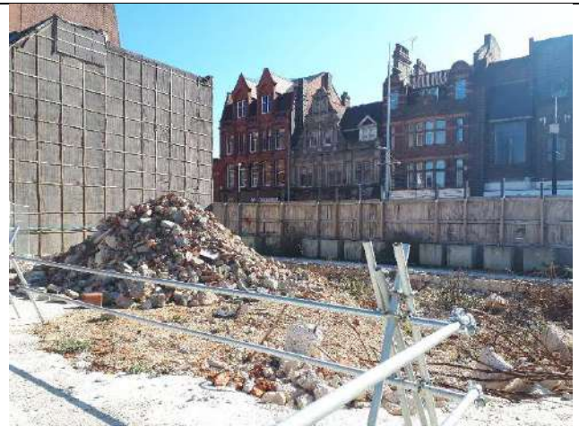
Photo 4 – View of stockpile containing broken out concrete in the south of the site – at higher topography than remainder of site.
