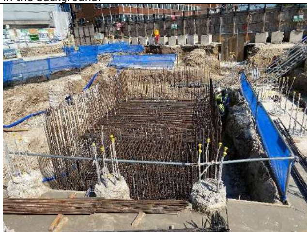
Photo 3 – Concrete core base in progress in the north west of the site (awaiting concrete pour).
