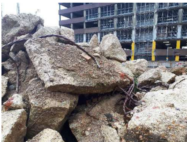
Photo 11 – Concrete and rebar stockpile in north east corner of site
