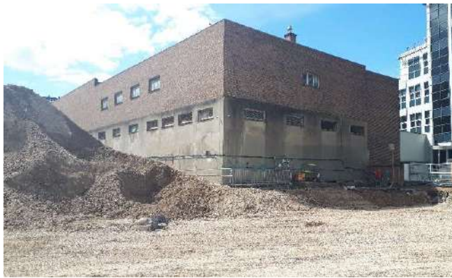
Photo 1 – Underpinning works complete beneath Sainsbury's building along the western site boundary.
