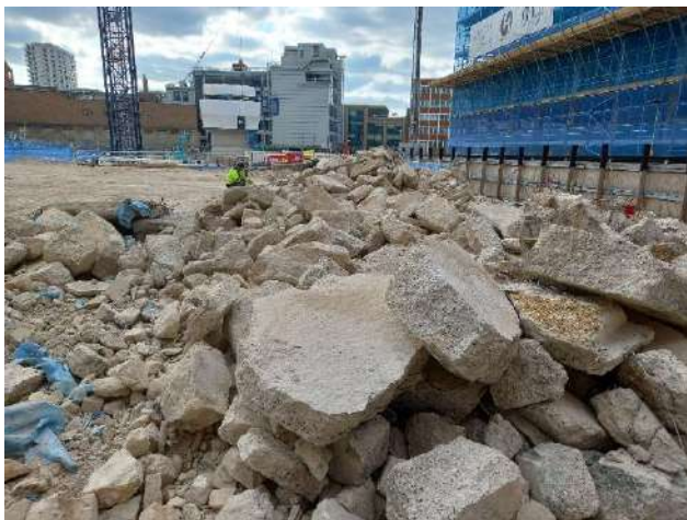
Photo 13 – Concrete slab and obstructions broken out in the far north east of the site. Ground beneath yet to be exposed.
