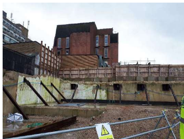
Photo 10 – Retaining wall in north east of the site
