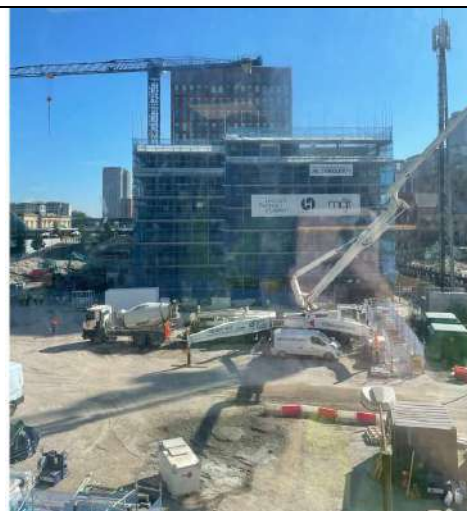
Photo 8 – View of the adjacent north site – demolition of the NCP car park being undertaken at the same time.
