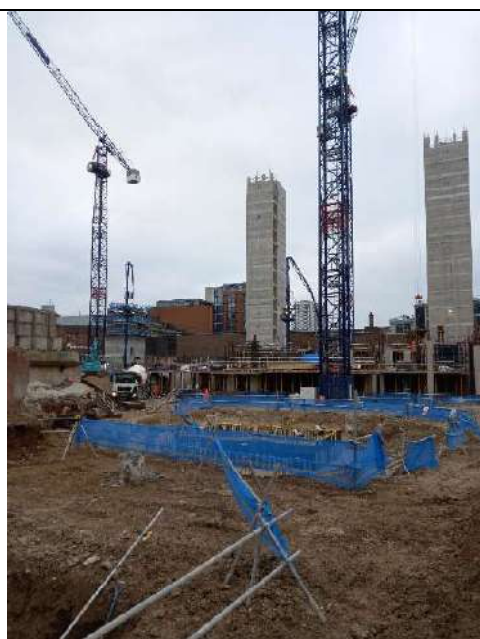
Photo 3 – View looking south across site, with cranes and building cores visible.
