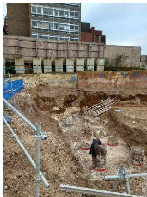
Photo 2 – Exposed piles adjacent to pile mat area in northeast corner.
