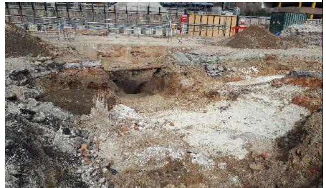
Photo 2 – View of concrete obstructions in the northern extent being broken out.
