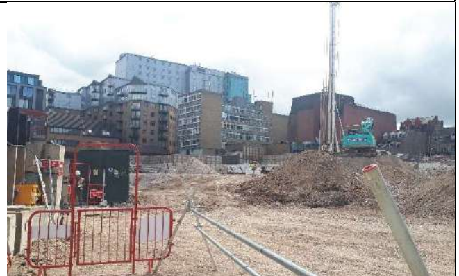
Photo 4 – View of piling rig in the centre of the site. Piling has not yet commenced (test piles undertaken over a year ago).
