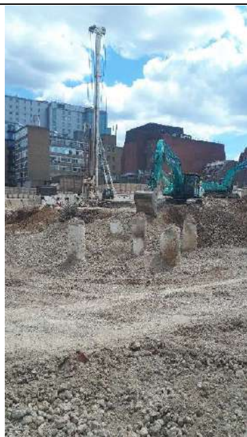
Photo 7 – Piling rig and exposed test piles located in the centre of the site.
