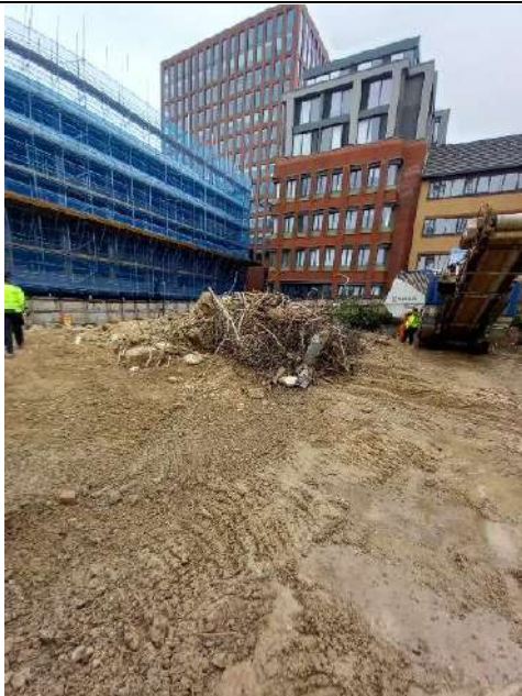
Photo 5 – Stockpile of metal rebar located in the northeast of site awaiting removal/disposal.
