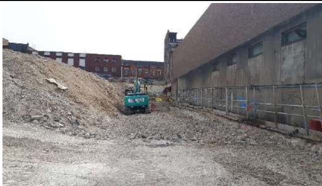
Photo 3 – Underpinning works being completed beneath the Sainsburys building located on the western site boundary.
