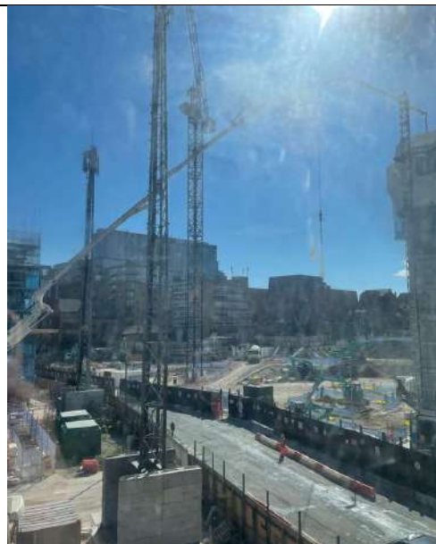
Photo 6 – View across the south site from Xfinity House site offices
