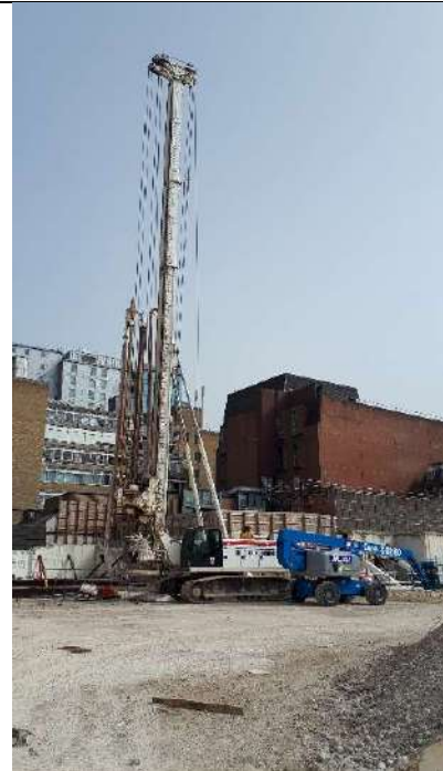
Photo 6 – View of piling rig in the centre of the site, which to date has undertaken approx. 20 test piles.
