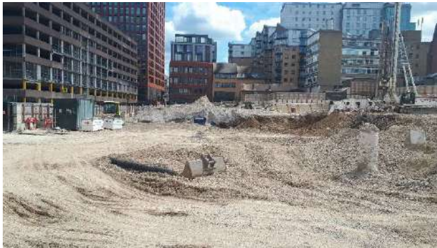
Photo 1 – View facing eastwards across the site showing the north western section now at formation level.
