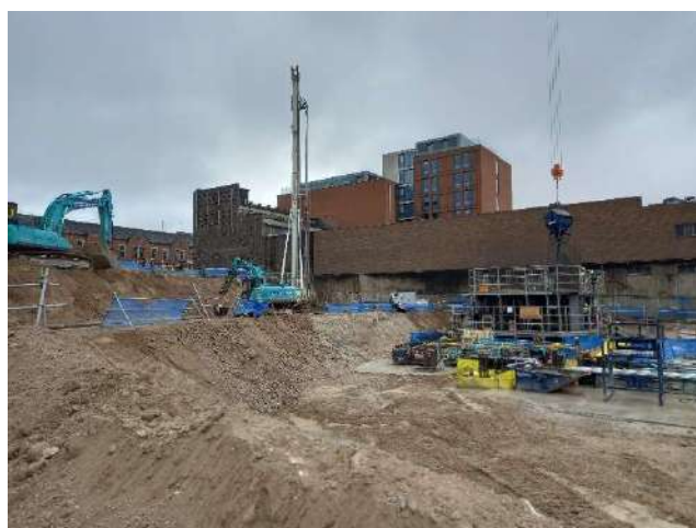
Photo 3 – View of the centre west showing ongoing piling at intermediate platform level.
