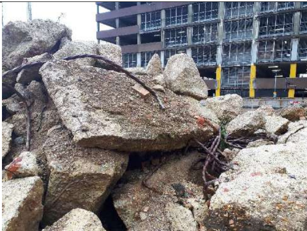
Photo 7 – Concrete and rebar stockpile in north east corner of the site
