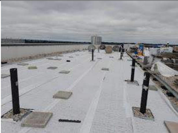
Photo 8 – Area due to form a green roof on level 12 of Block E.
