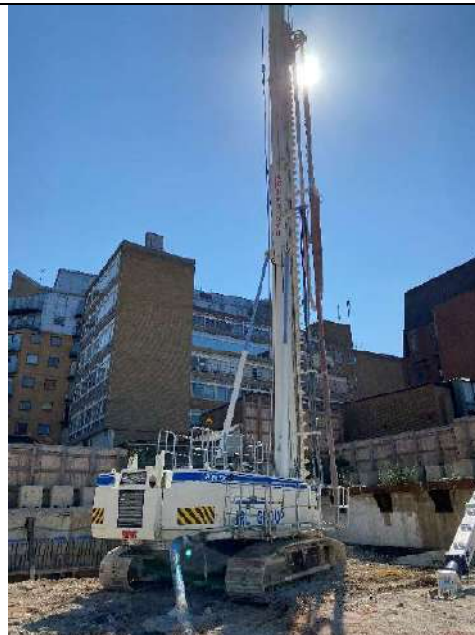
Photo 6 – Piling rig in operation adjacent to the retaining wall on the eastern site boundary.
