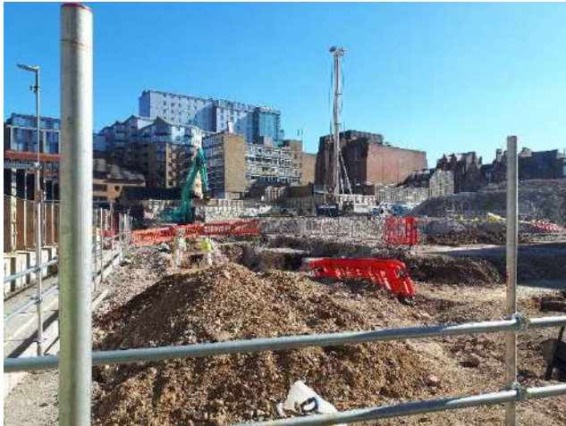
Photo 1 – View across site facing east (from north west corner) and north western archaeology pit
