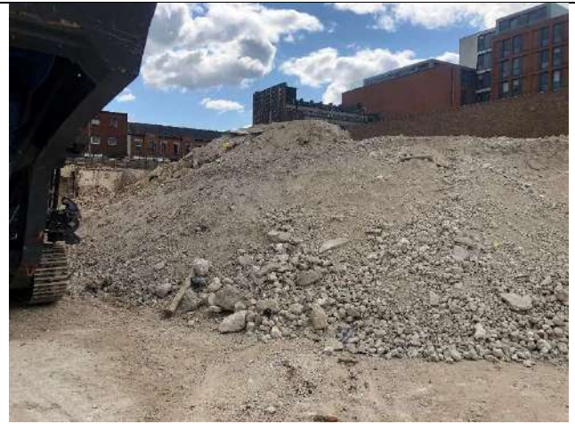
Photo 8 – Stockpile of crushed concrete to be removed from site.
