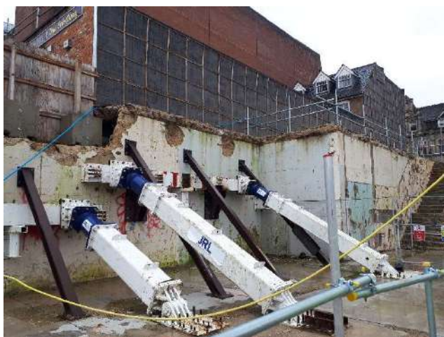
Photo 5 – Retaining wall along eastern boundary
