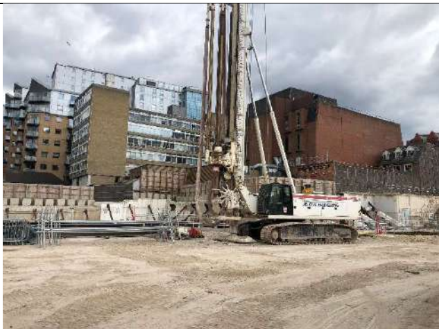
Photo 3 – View of piling rig set up (previously installed test piles only).
