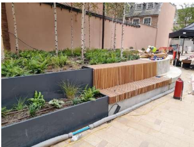
Photo 3 – Soft landscaping in Friars Walk.
