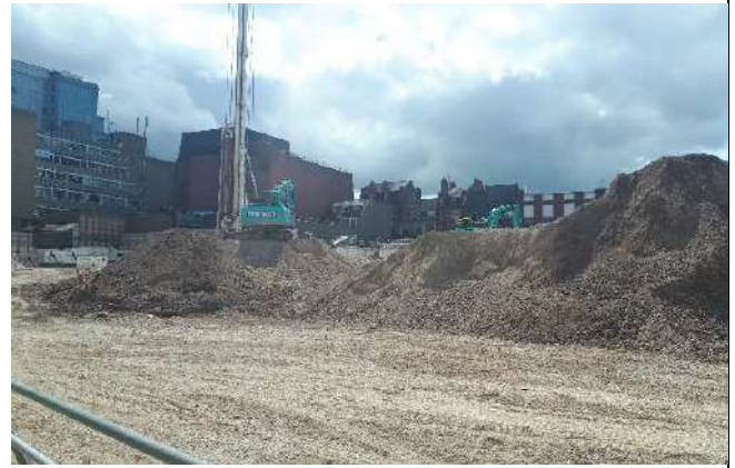
Photo 2 – View across site from north west showing north western area at formation level.
