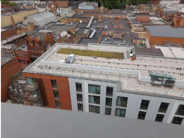
Photo 5 – View of green roof on top of level 6 (south of Block E)
