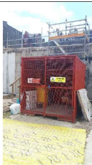
Photo 8 – Secured COSHH cabinet located in the south of the site.
