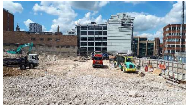
Photo 2 – View facing westwards across the north of the site showing north western section now at formation level.
