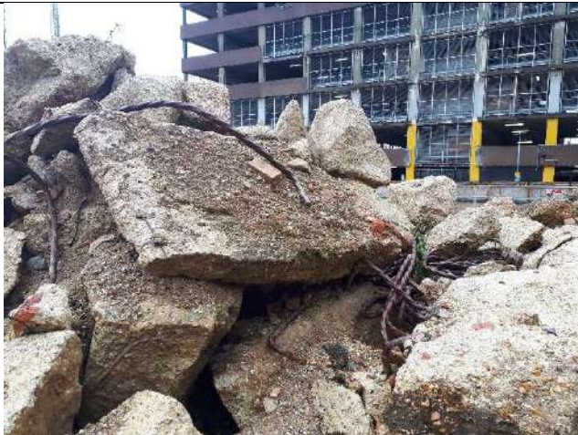
Photo 7 – Concrete and rebar stockpile in north east corner of south site
