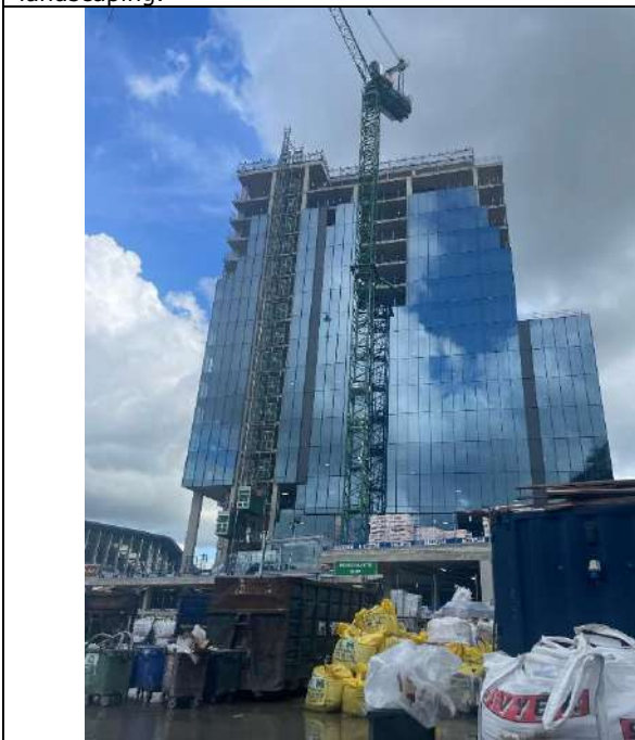
Photo 11 – View of new building to the east of North Site.
