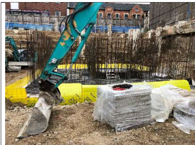
Photo 1 – Block E southern core excavated and installed.
