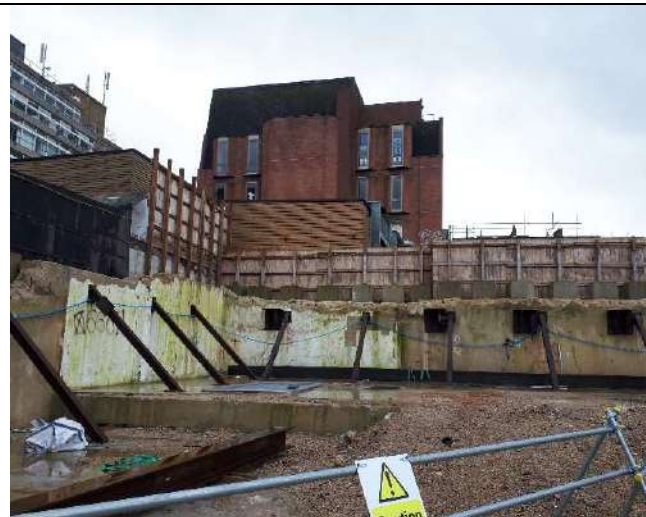
Photo 6 – Retaining wall in north east of the site
