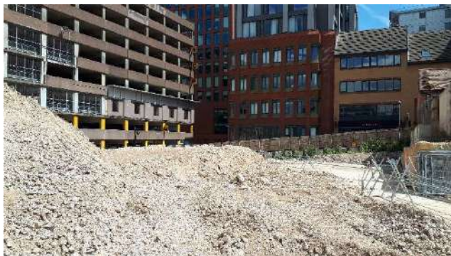
Photo 5 – Stockpiles of concrete crush currently stored within the north east of the site.
