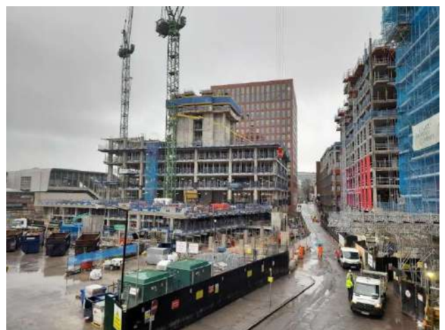
Photo 4 – Excavations of Garrard Street scheduled for February 2023.
