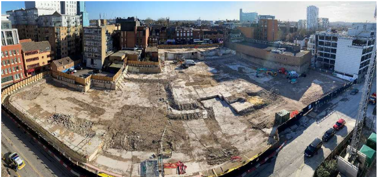
Photograph of the South Site post demolition
