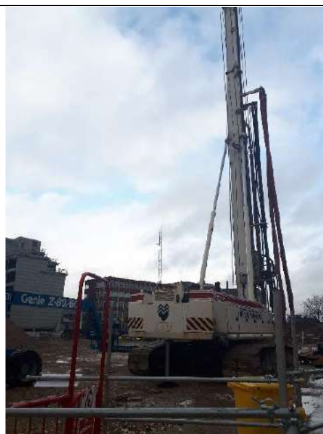
Photo 12 – Piling rig on concrete slab in the centre of the site
