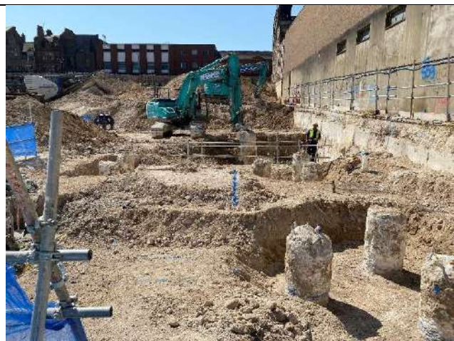
Photo 4 – View along the western site boundary. Excavations and breaking out of pile caps in progress.
