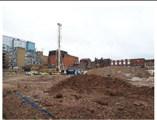
Photo 2 – View across the site facing south east
