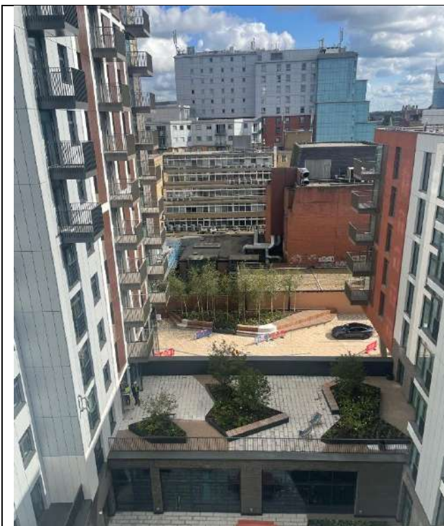
Photo 9 – View of communal area completed soft landscaping.
