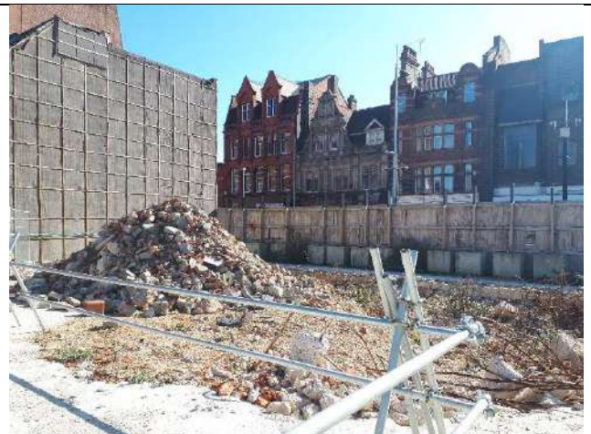
Photo 4 – View of stockpile from broken out concrete in the south of the site – at higher topography than remainder of site.
