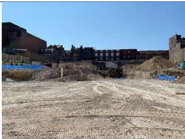
Photo 1 – View facing south across the centre of the site (at formation level). Stockpiles of demolition crush present in the background.
