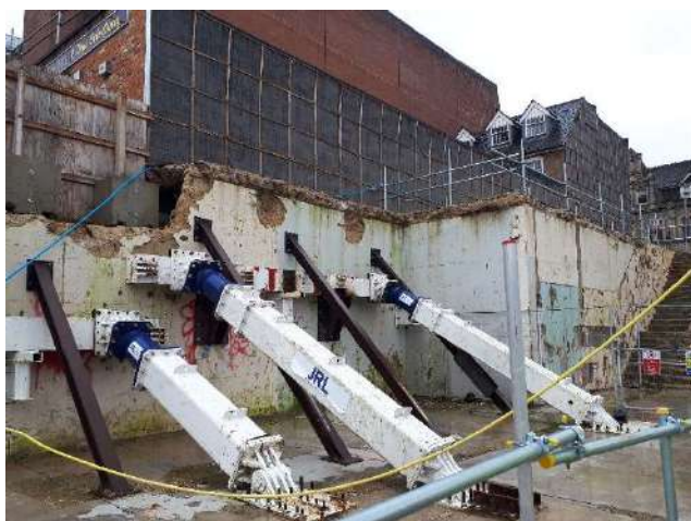
Photo 9 – Retaining wall along eastern boundary
