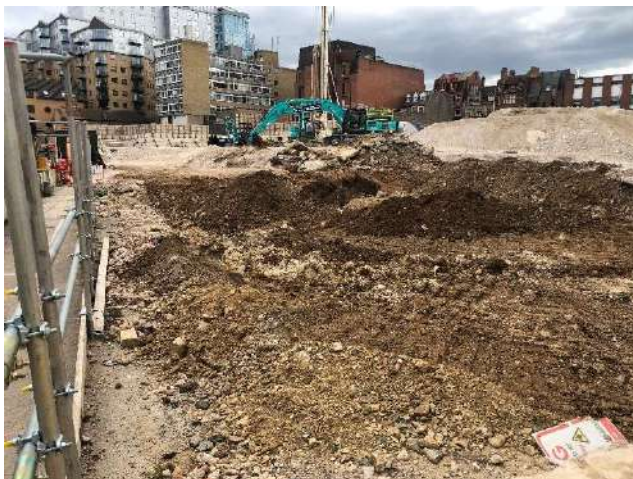
Photo 1 – View across site facing east (from north west corner) and north western archaeology pit (concrete and brick obstructions are being removed).
