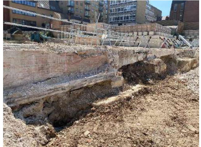
Photo 6 – Close-up view of the concrete slab in place in the north eastern section of the site.
