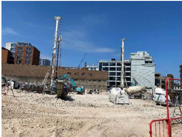
Photo 1 – View facing westwards across the site showing the north western section now at formation level and a piling rig in progress.
