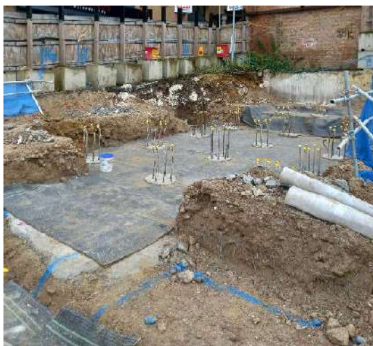
Photo 1 – Northeast corner of site with pile caps installed
