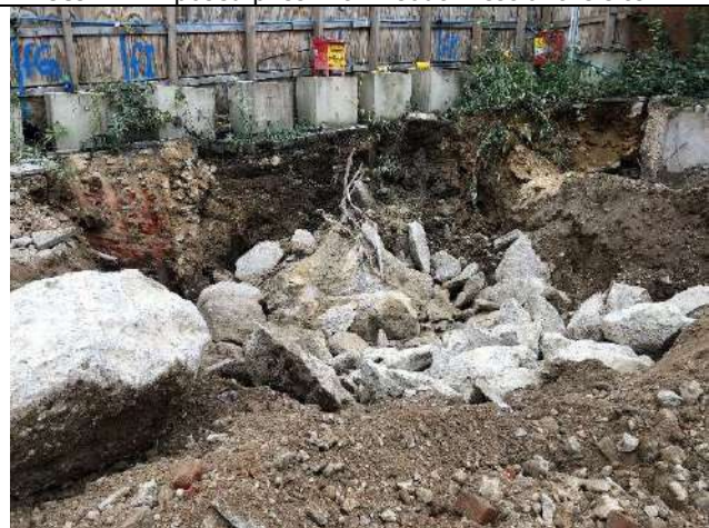
Photo 4 – Last remaining concrete obstruction within the northeast corner of site awaiting excavation.
