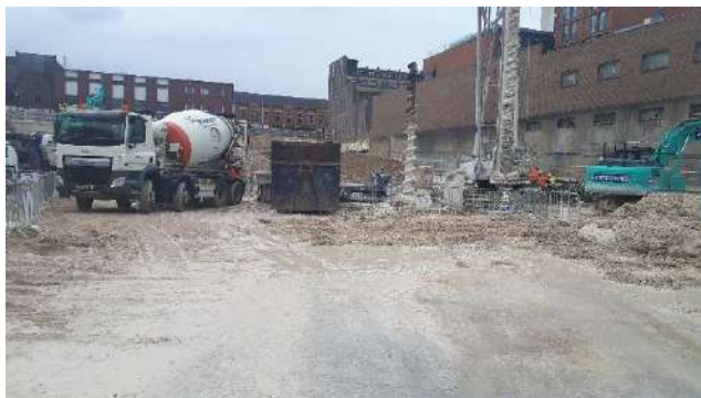
Photo 3 – View facing south west across site showing second piling rig in central west.
