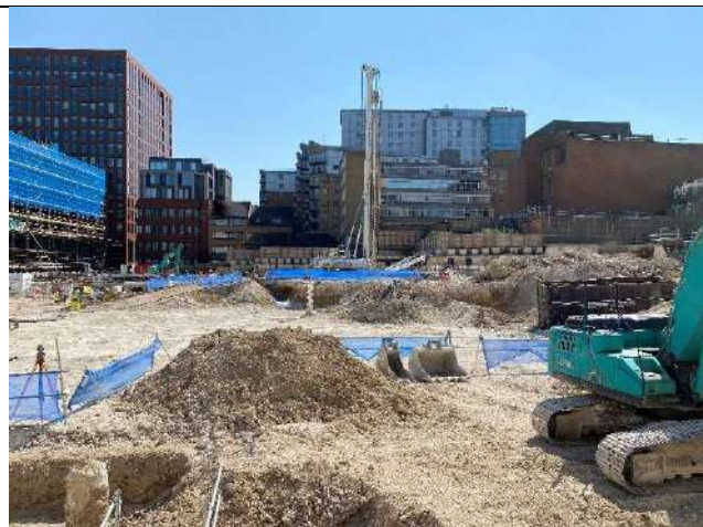
Photo 2 – View facing east across the site.
