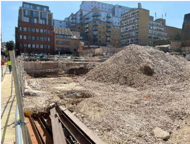
Photo 5 – Viewing facing eastwards, showing the concrete slab in place in the north western section of the site. Stockpiles of concrete crush are currently stored within the northeast of the site.
