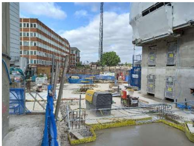
Photo 3 – View of the concrete slab in the north west corner of the site. The new sub station and services to be installed here.
