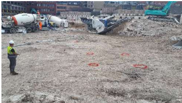
Photo 1 – View of centre west of site at formation level with piling works complete.
