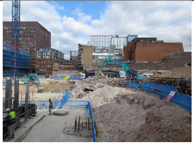
Photo 8 – View facing east across the central area of the site.
