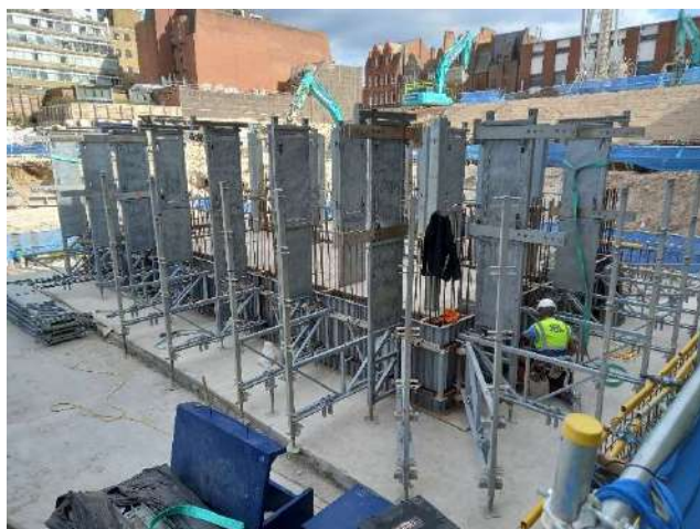
Photo 5 – Slip form under construction on the core in the west of the site.
