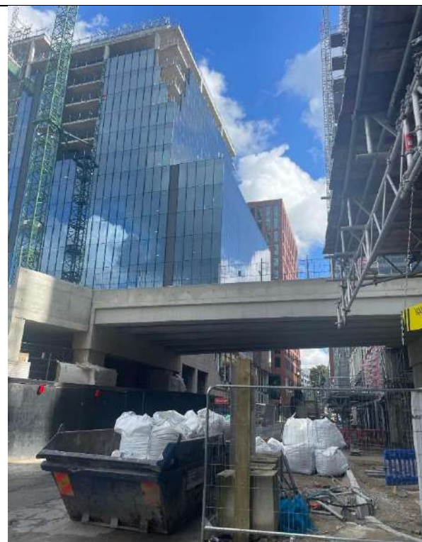
Photo 10 – New walkway over Garrard Street.
