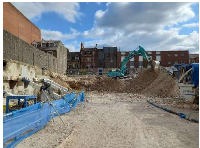
Photo 10 – View along the eastern site boundary, concrete slab yet to be broken out.
