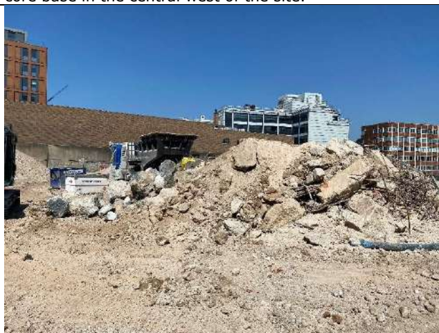
Photo 7 – Stockpile of demolition material comprising concrete slabs and rebar, crusher present in the background.
