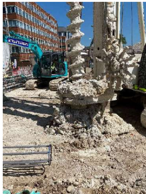
Photo 10 – Close-up view of the material being removed during the drilling of piles.
