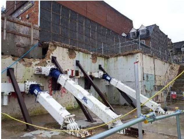
Photo 5 – Retaining wall along eastern boundary
