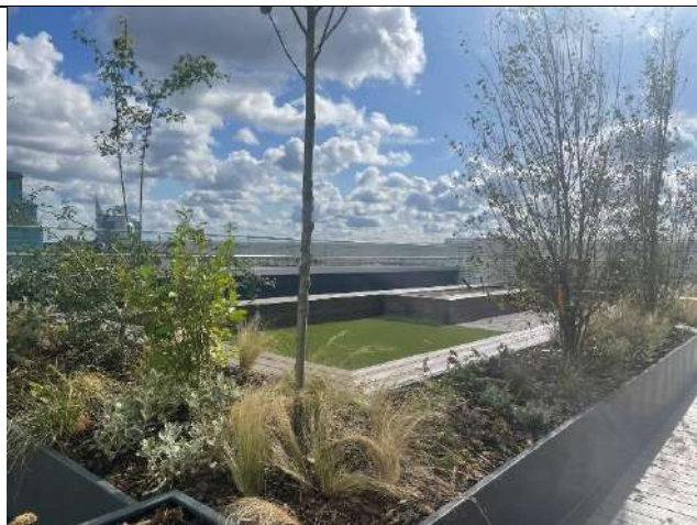
Photo 5 – View of green roof on Level 7.
