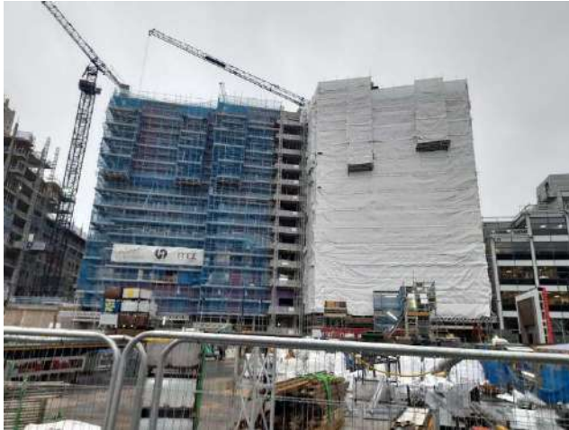
Photo 1 – View of Phase 1 from Phase 2.
