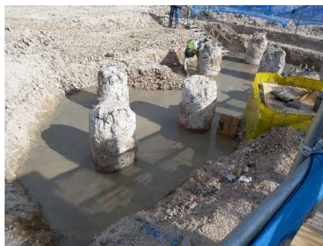
Photo 6 – Excavation to expose pile caps, binding concrete poured.
