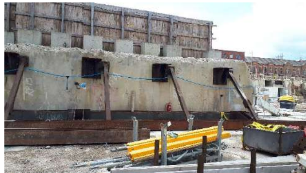
Photo 6 – Retaining wall in north east of the site
