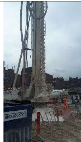
Photo 4 – Piling being undertaken in central north of the site forming a chalky slurry.
