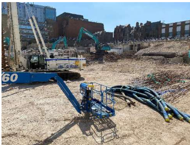
Photo 3 – View facing south east across the central area of the site, showing excavators moving and stockpiling crushed material. Concrete slabs and obstructions are noted in the south of the site.
