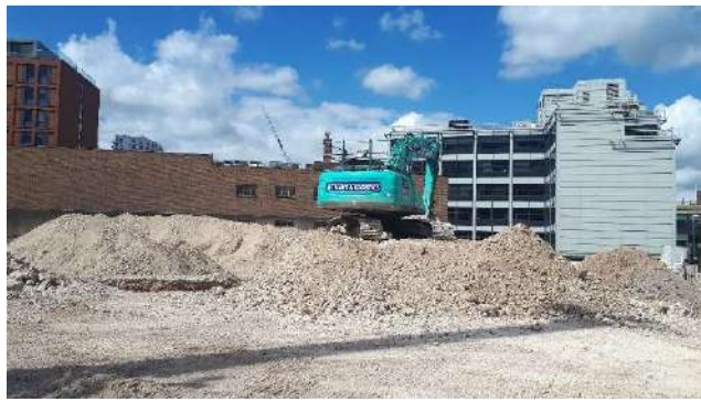
Photo 3 – Stockpiles of concrete crush in the centre of the site.
