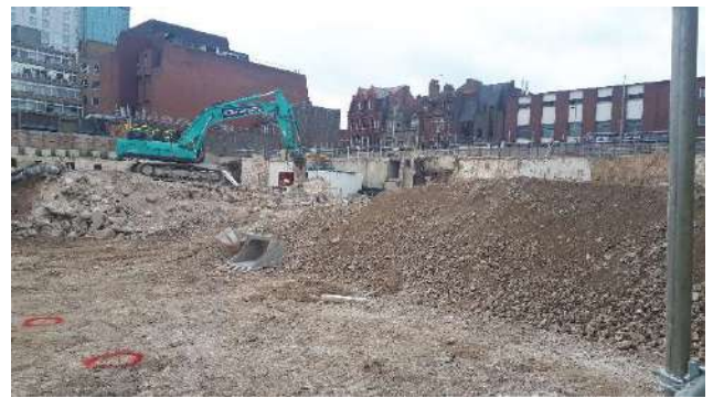
Photo 2 – View facing south east across the site showing stockpiles of excavated material and concrete being broken out in the east.
