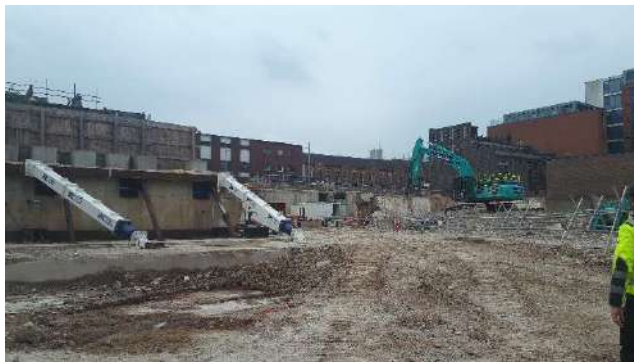
Photo 5 – North east of south site where concrete breakout and excavations have not yet commenced. Eastern boundary retaining wall is visible.
