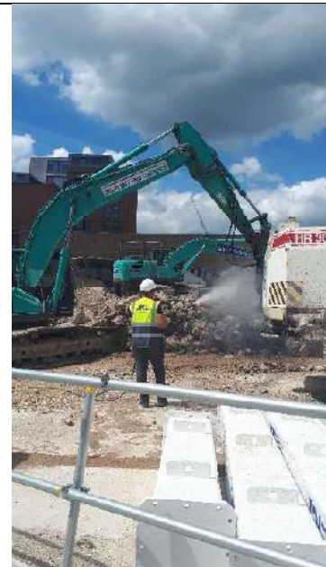
Photo 4 – Dampening down of stockpiles being undertaken during concrete breakout and crushing works.
