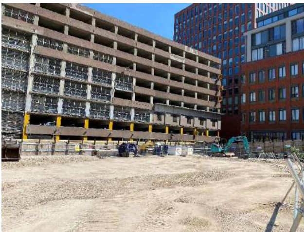
Photo 7 – View of the north eastern area of the site, where the concrete slab is still in place.
