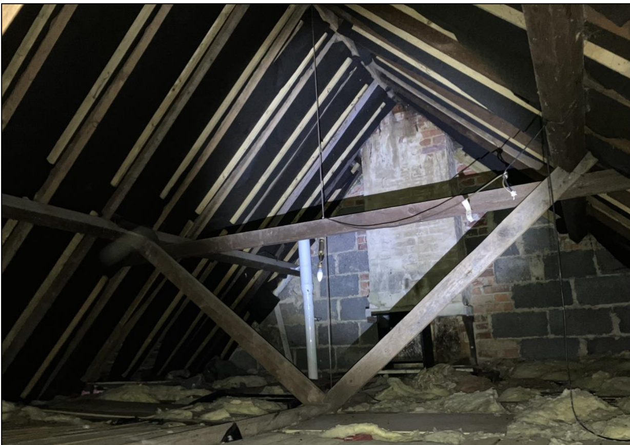
Photograph 4. The loft space within the roof of the dwelling.
