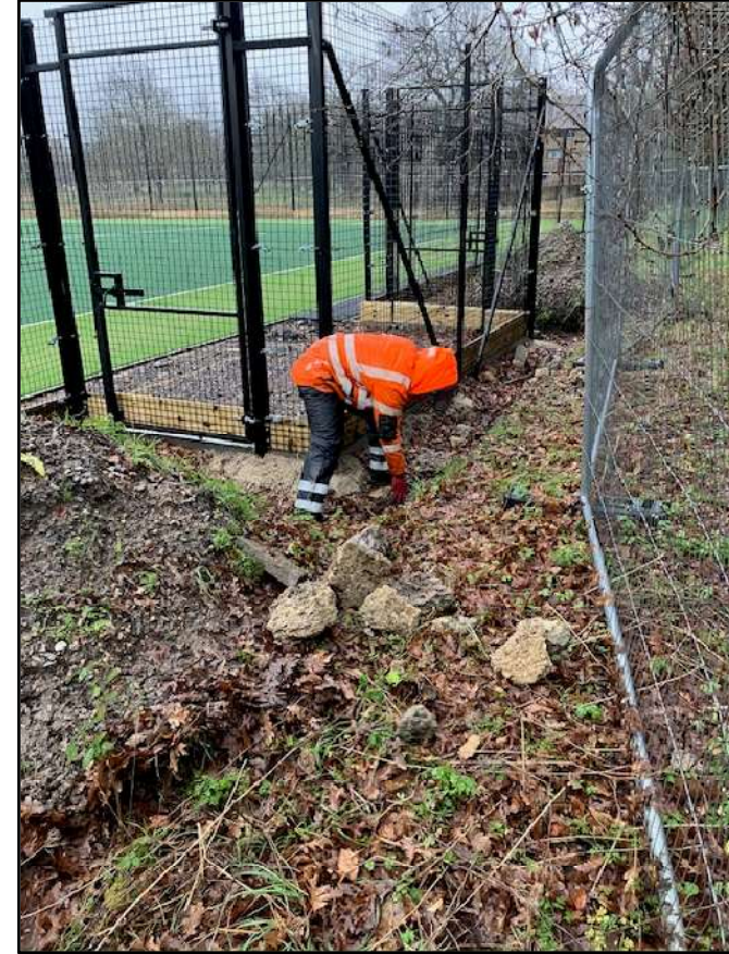
Figure 3: T1 Oak. Removal of excess spoil including broken out concrete haunching.
