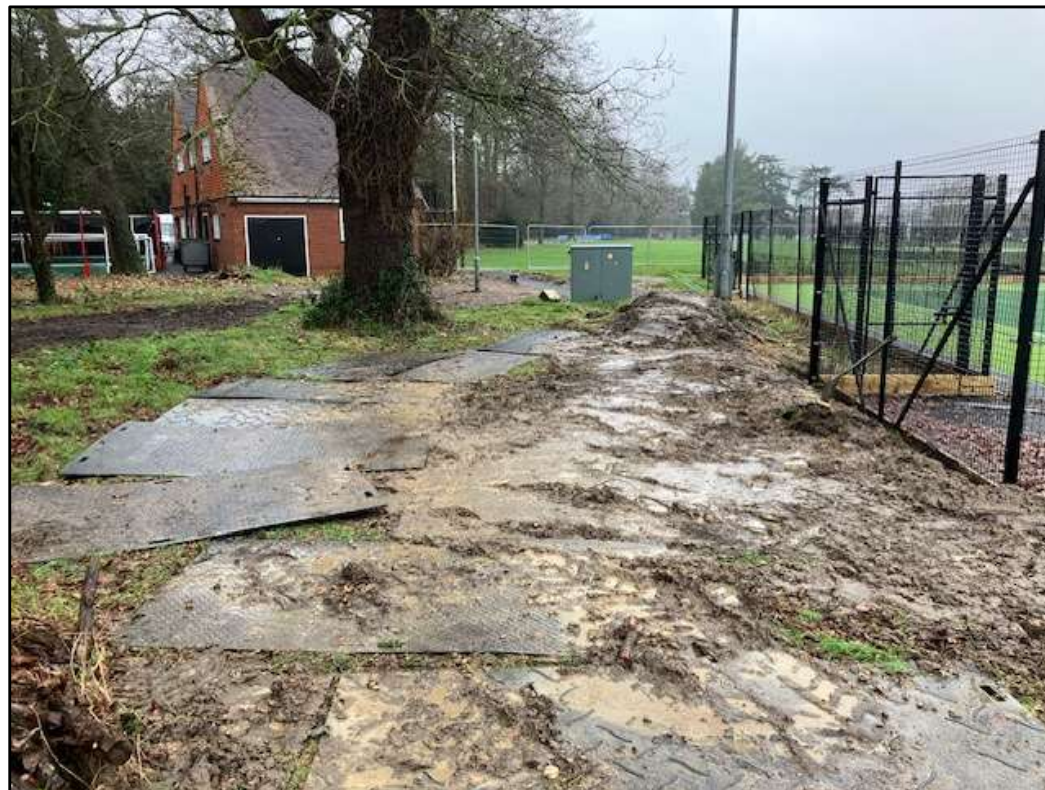
Figure 8: T9 Oak. Removal of excess spoil. Utilisation of Ground Mats.:
