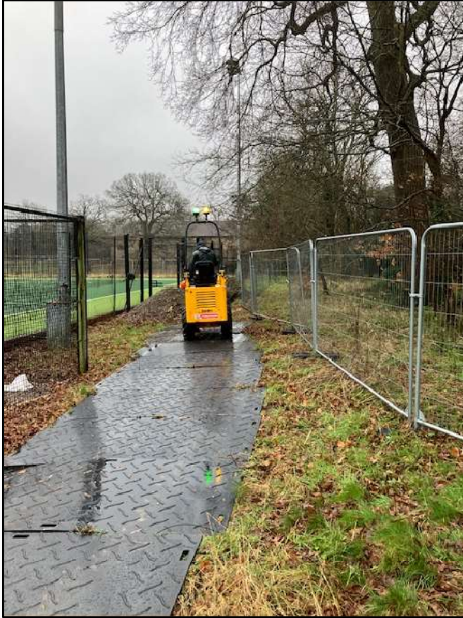
Figure 2: T1 Oak. Removal of excess spoil. Utilisation of Ground Mats.
