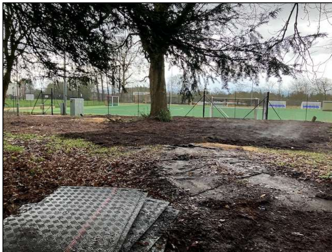
Figure 10: T1 Oak. Installed topsoil conditioner and composted woodchip mulch.
