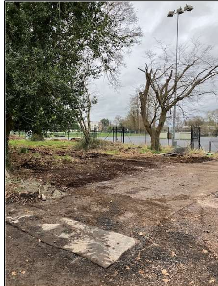
Figure 12.: Mound of construction stone removed from within the RPA's of trees within TPO Area W4.
