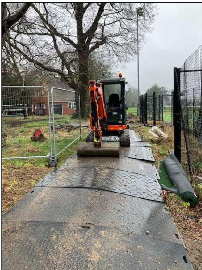
Figure 7: T9 Oak. Removal of excess spoil. Utilisation of Ground Mats.
