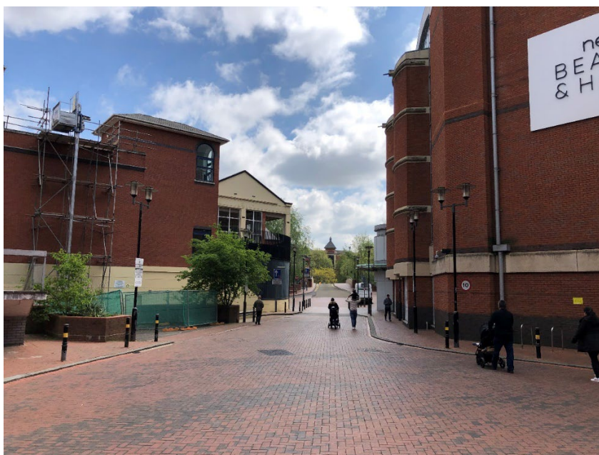
Figure 8.8 View looking south along Yield Hall Place and bridge to the east side of the Site
