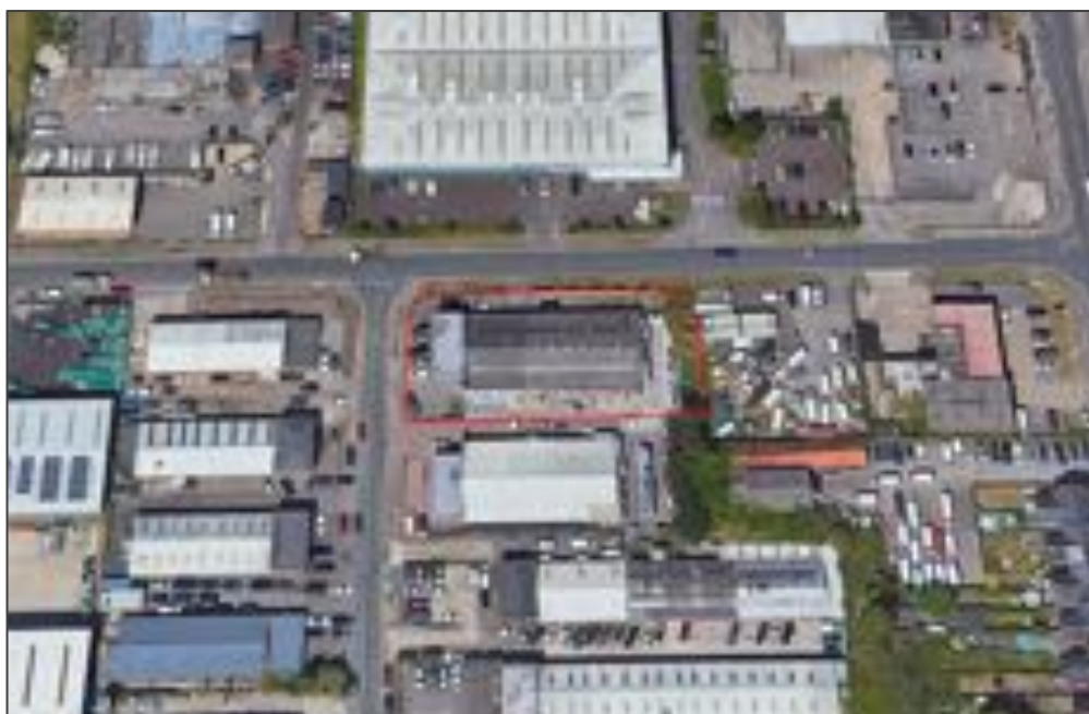
Figure 1: Approximate location of the red line boundary.
