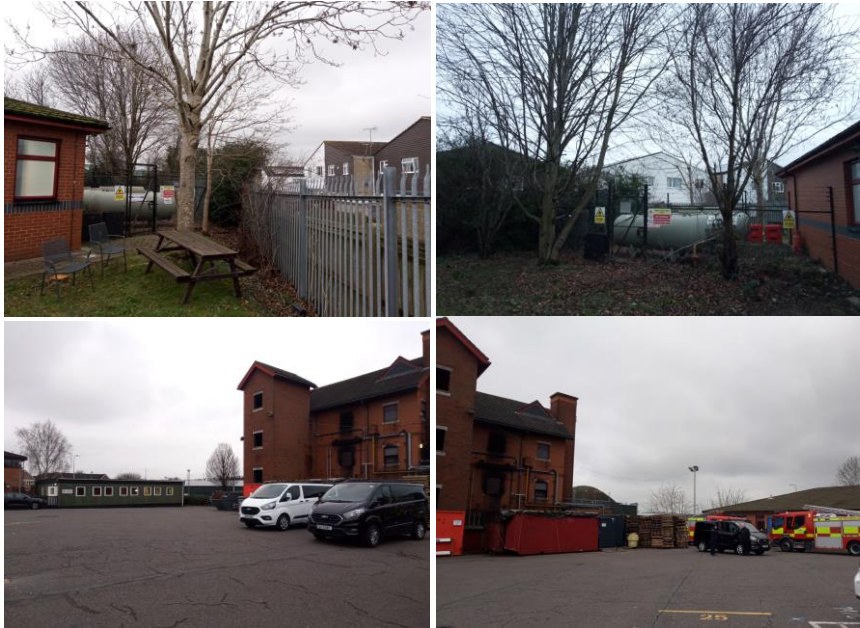
Temporary building to be demolished
