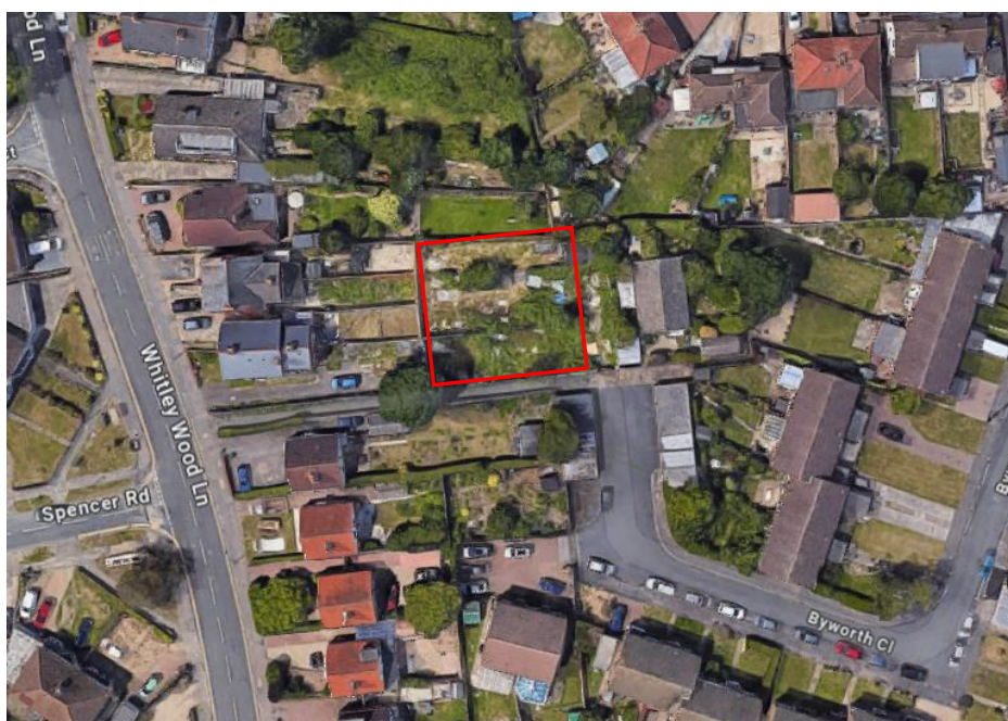
Aerial view of the application site (outlined in red) taken from Google Maps on 12/03/2024.
