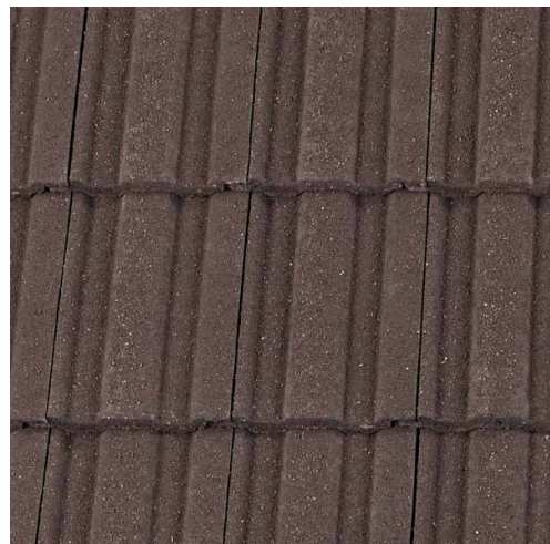
Existing Roofing Material
