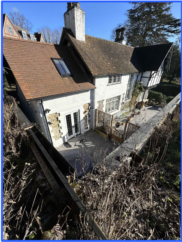
RETAINING WALL TO BE LOWERED AND RECONSTRUCTED WITH BRICK AND FLINT FACADE
