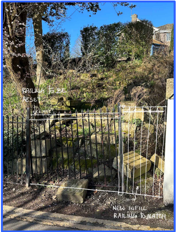
PROVIDE INFILL METAL RAILING TO MATCH
