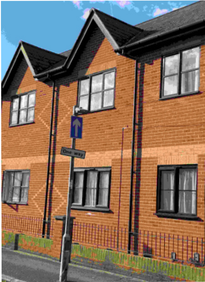
Figure 15 Flatted development, Queens Road March 2024
