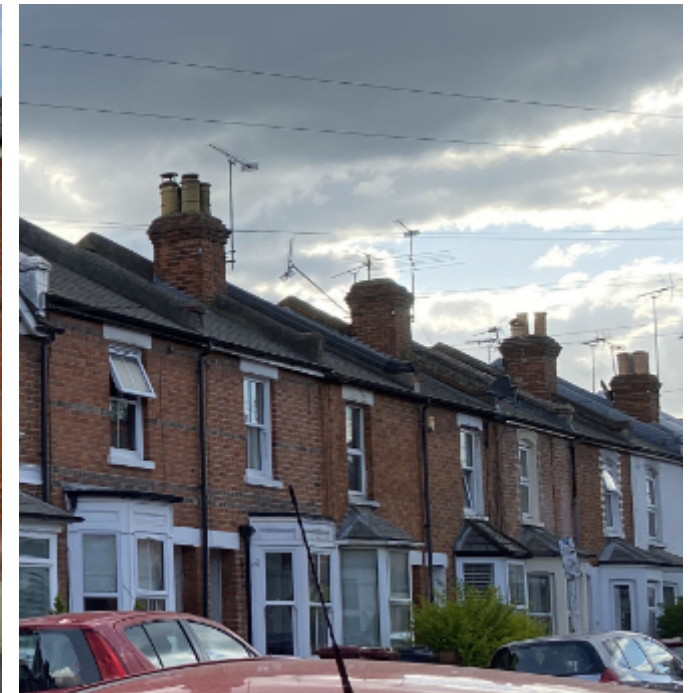
Figure 9 Raised party wall parapets & chimneys along Queens Road
