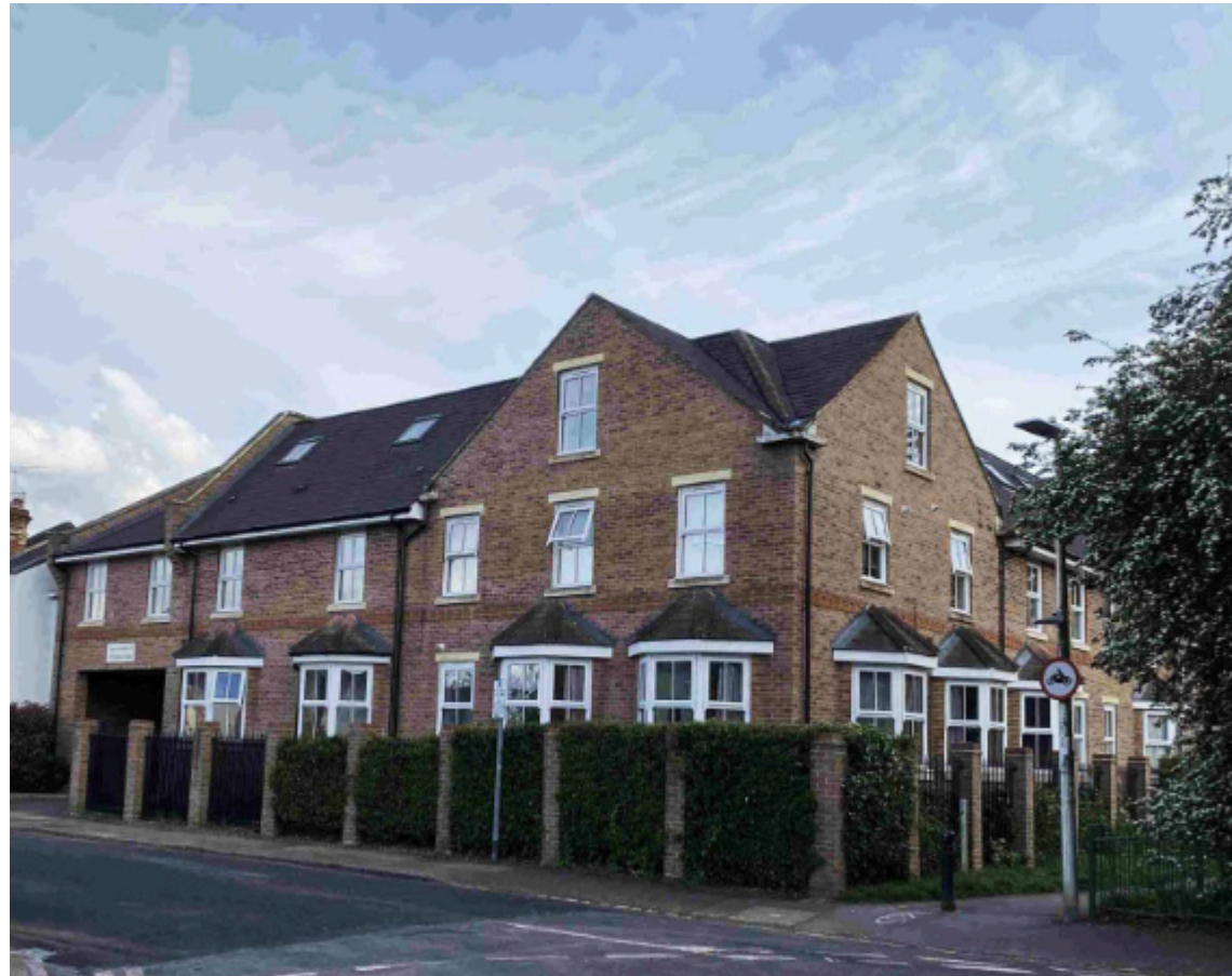
Figure 14 Flatted development, no 129 Queens Road
