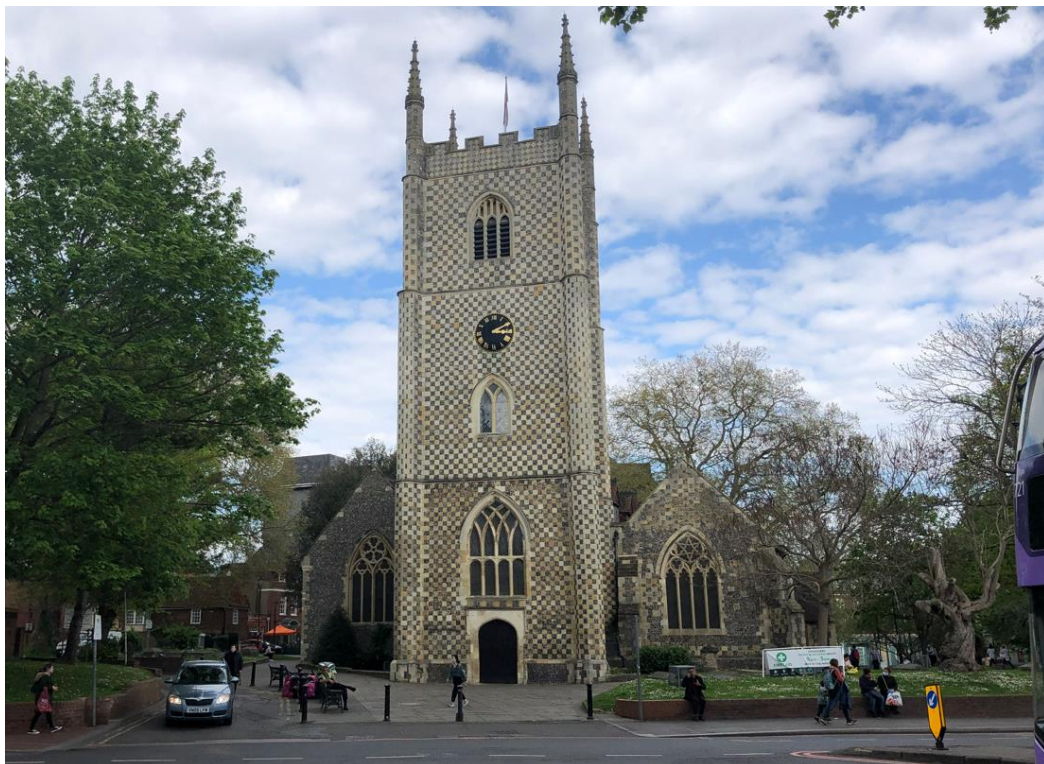
Figure 5.31: View of Church of St Mary's and its Churchyard
