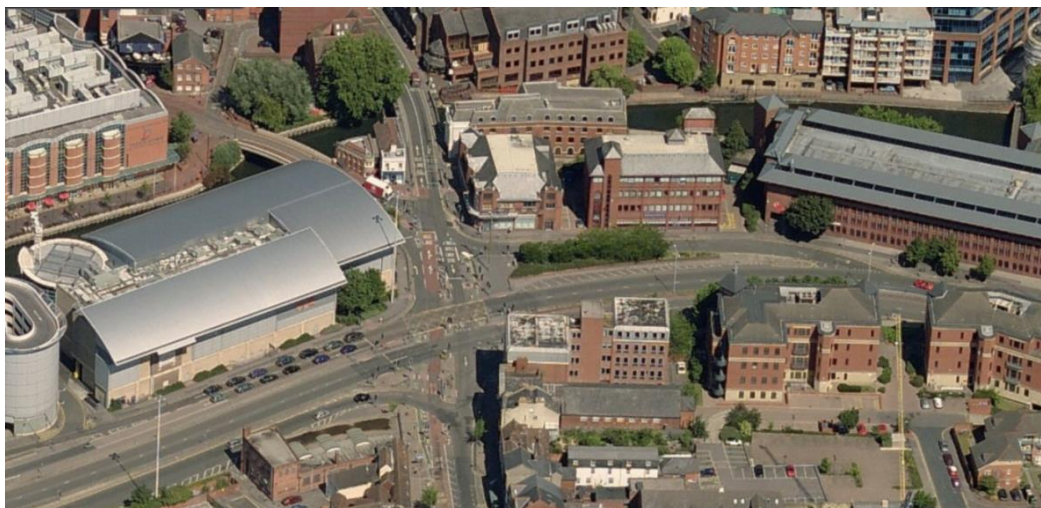
Figure 5.24: Area 3: Contrasting larger scale modern development dilutes the historic character of this part of the conservation area
