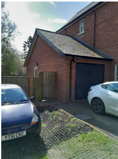
Property: front elevation with side access.
