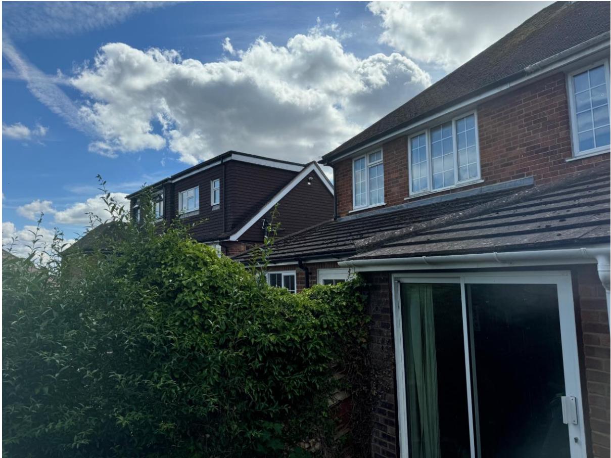
Site Visit photos taken on 11 th of July 2024
