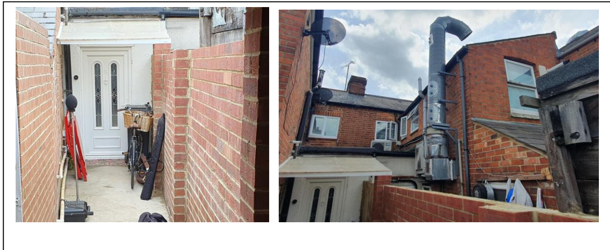
Figure 3: Site Location Measurement Pictures
