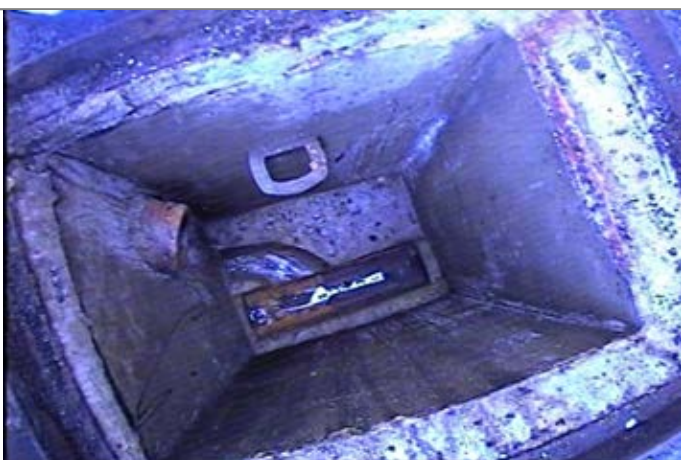
Manhole / Access Point: SWMH12 Internal
