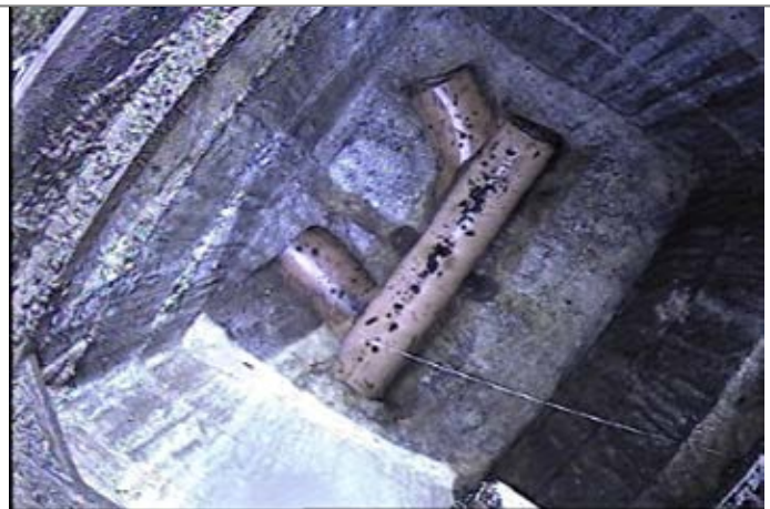
Manhole / Access Point: FWMH13 Internal
