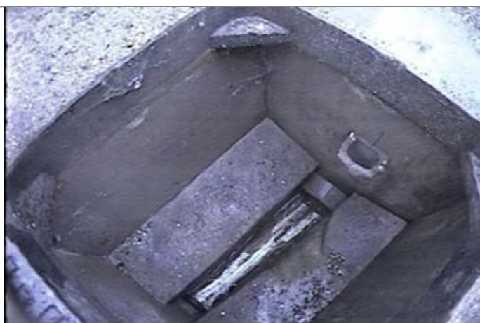
Manhole / Access Point: FWMH2 Internal
