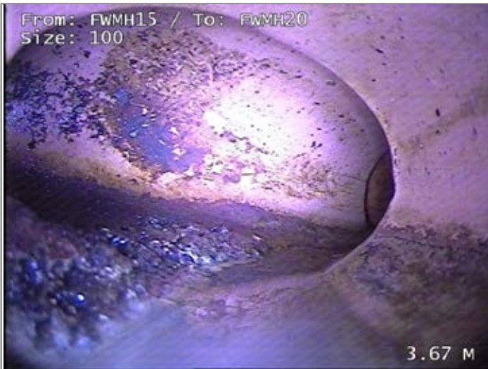
JOINING ANOTHER PIPE
