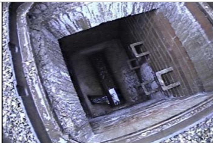
Manhole / Access Point: SWMH5 Internal
