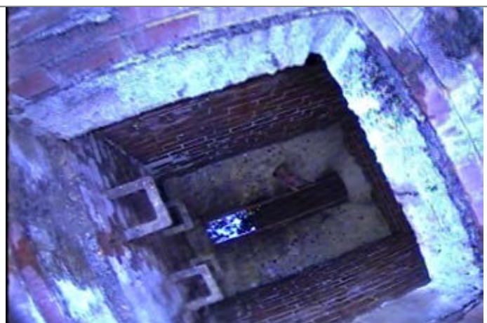
Manhole / Access Point: SWMH14 Internal
