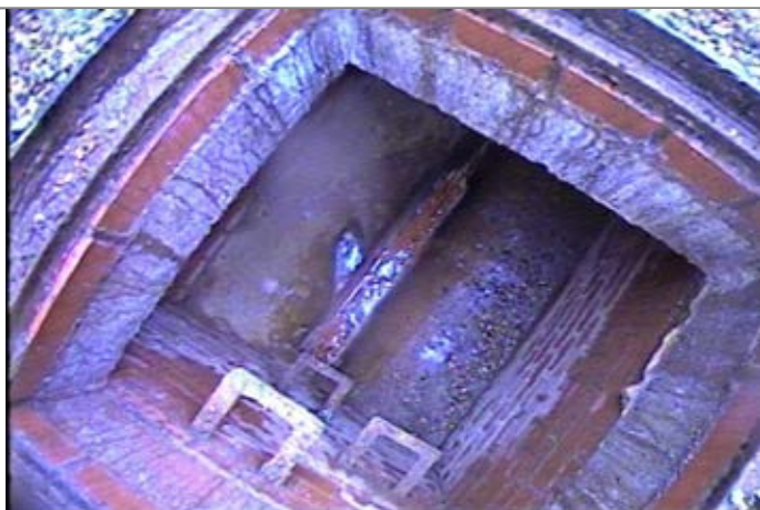
Manhole / Access Point: SWMH2 Internal
