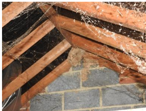
Fig. 26 Cobwebbed gable end
