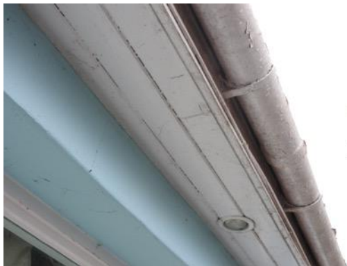
Figs. 20 & 21 Tightly fitting boxed soffits against the walls
