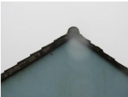
Figs. 17 & 18 Sealed gables to the north and southeast
