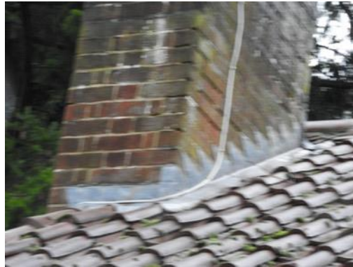
Fig. 14 Tightly moulded lead flashing
