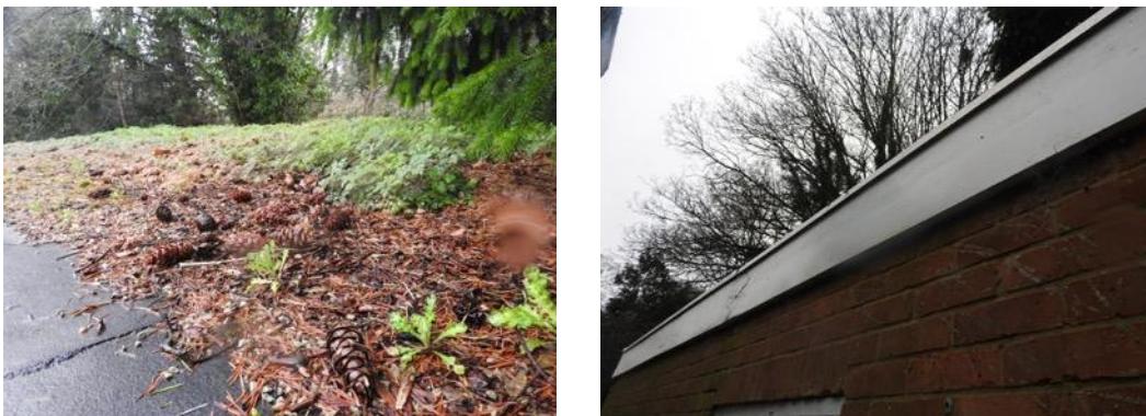
Figs. 27 & 28 Vegetation covered roof and tightly fitting timber fascia boards
