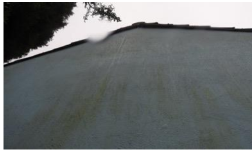
Fig. 19 Sealed gable to the east
