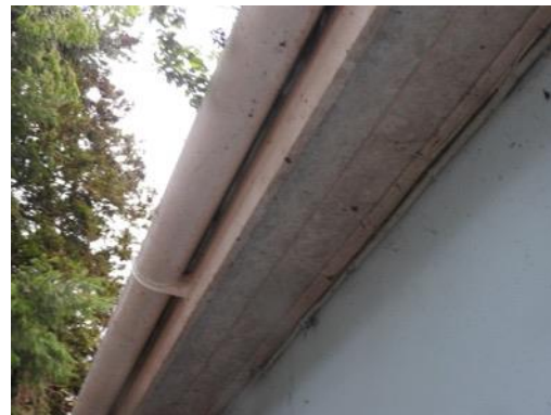
Figs. 20 & 21 Tightly fitting boxed soffits against the walls
