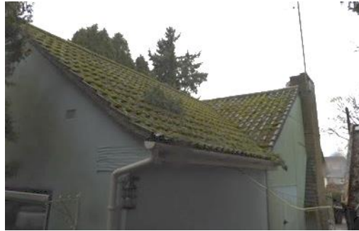
Fig. 7 Ridge and roof tiles to the west
