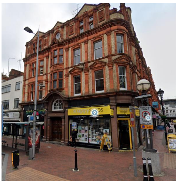
150 Friar Street as seen from Friar Street junction with Station Road and Queen Victoria Street.
