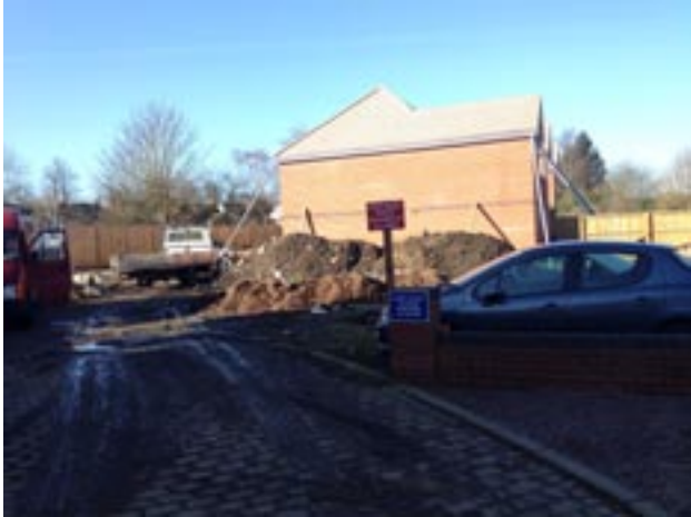
5 New residential development to the north west of the site, partially complete
