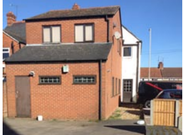
6 Rear of properties facing Norcot Rd, behind the site
