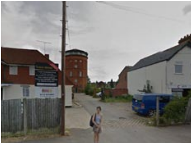
1 View from Norcot Road along the site access road with the Listed Water Tower.
