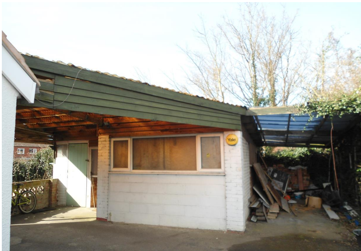
Fig 4: Outbuilding to the rear of 216 Whitley Wood Lane and boundary fence beyond
