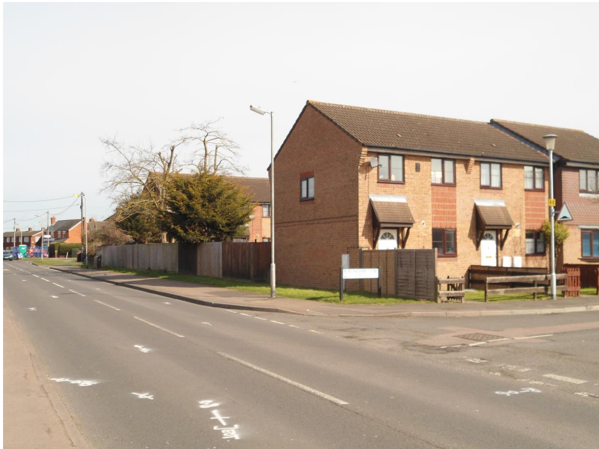
Fig 17:1 Burlingham Close Flank Wall leading to Whitley Wood Lane
