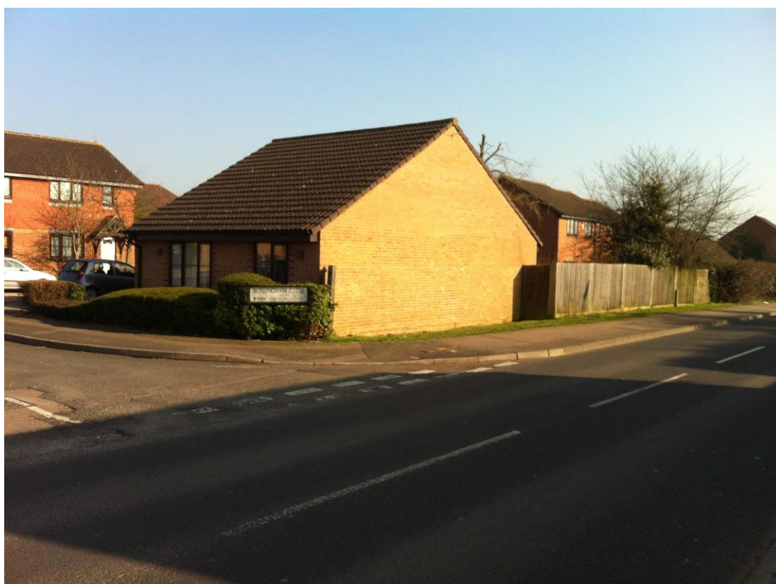
Fig 16: Flank wall of 4 Burlingham Close
