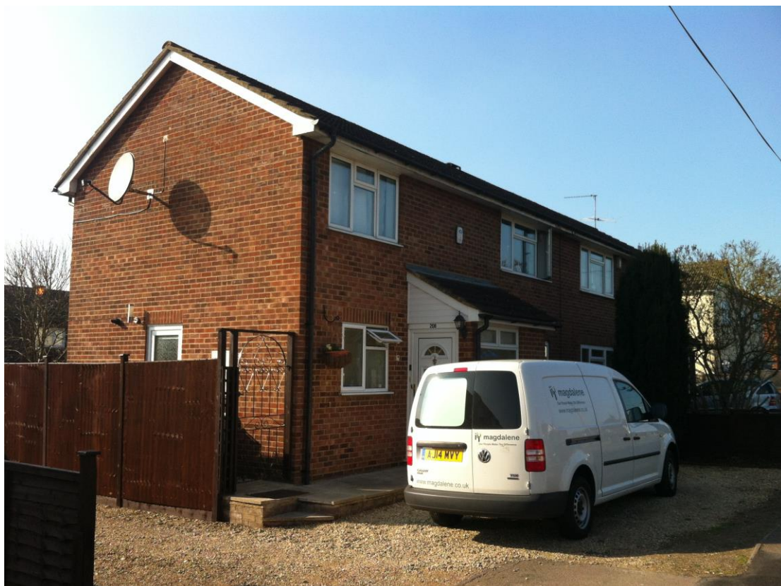
Fig 7: Gable Ended roof on Whitley Wood Lane
