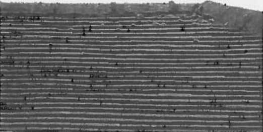
5. The tightly fitted flat, clay roof tiles.
