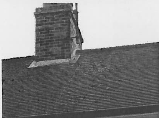
9. Tightly fitted lead flashing present around chimney.
