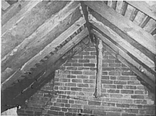
15. Lightly cobwebbed ridge beam and chimney present to the north.
