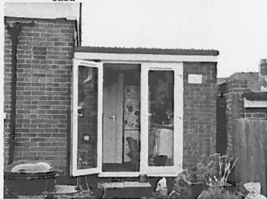
4. The single storey flat roofed extension to the south.
