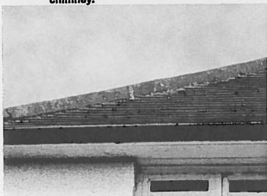
11. Tightly secured wooden soffit boxes.
