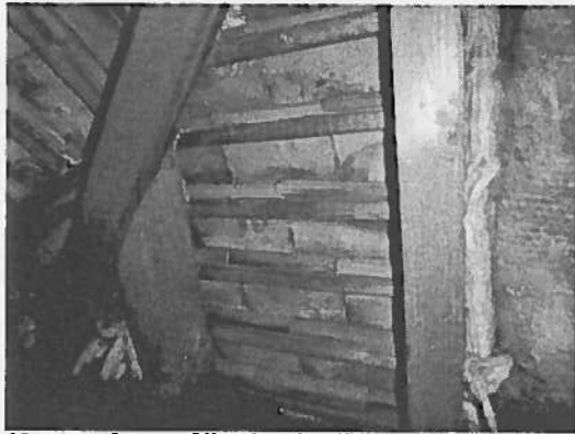
13. Areas of lined and unlined roofing tiles.
