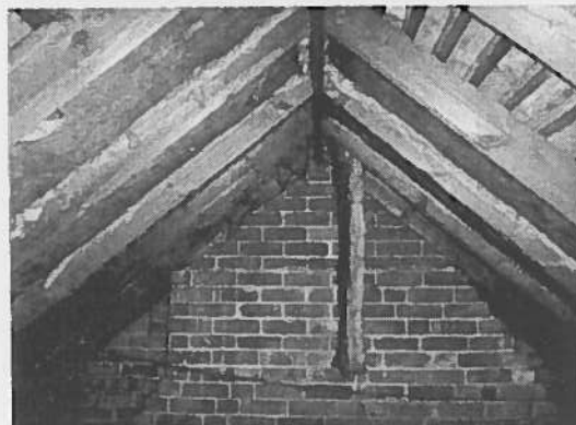
12. Cut and pitch roof construction within hipped roof space.
