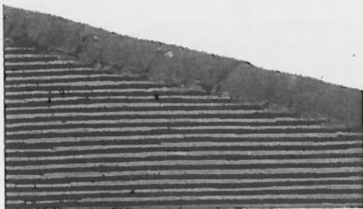
7. Tightly mortared ridge and hipped tiles.
