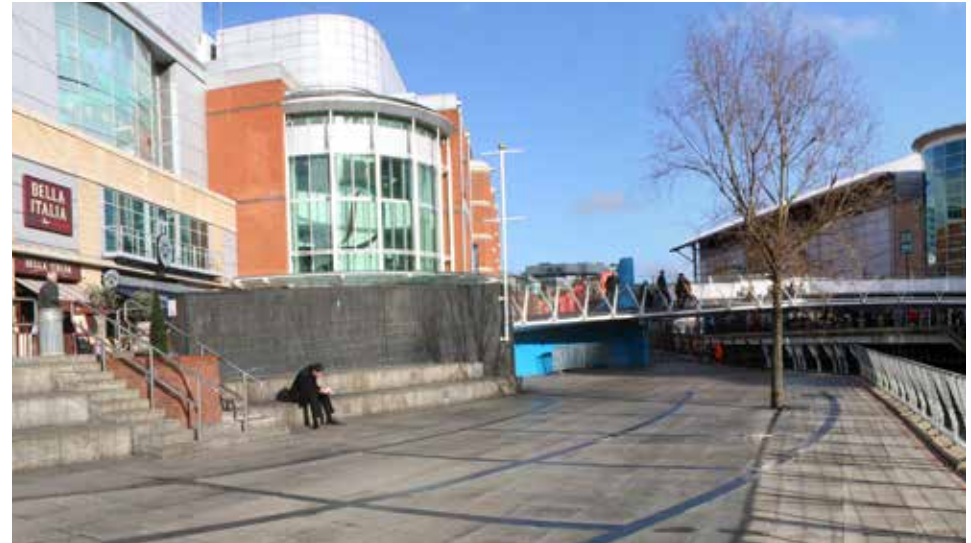
Area of North bank at Eastern bridge abutment
