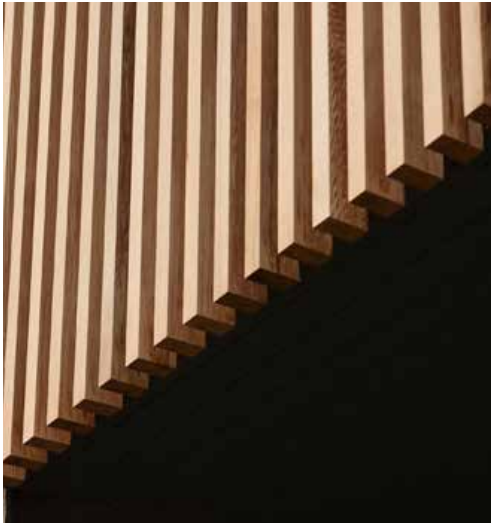
Vertical timber cladding
