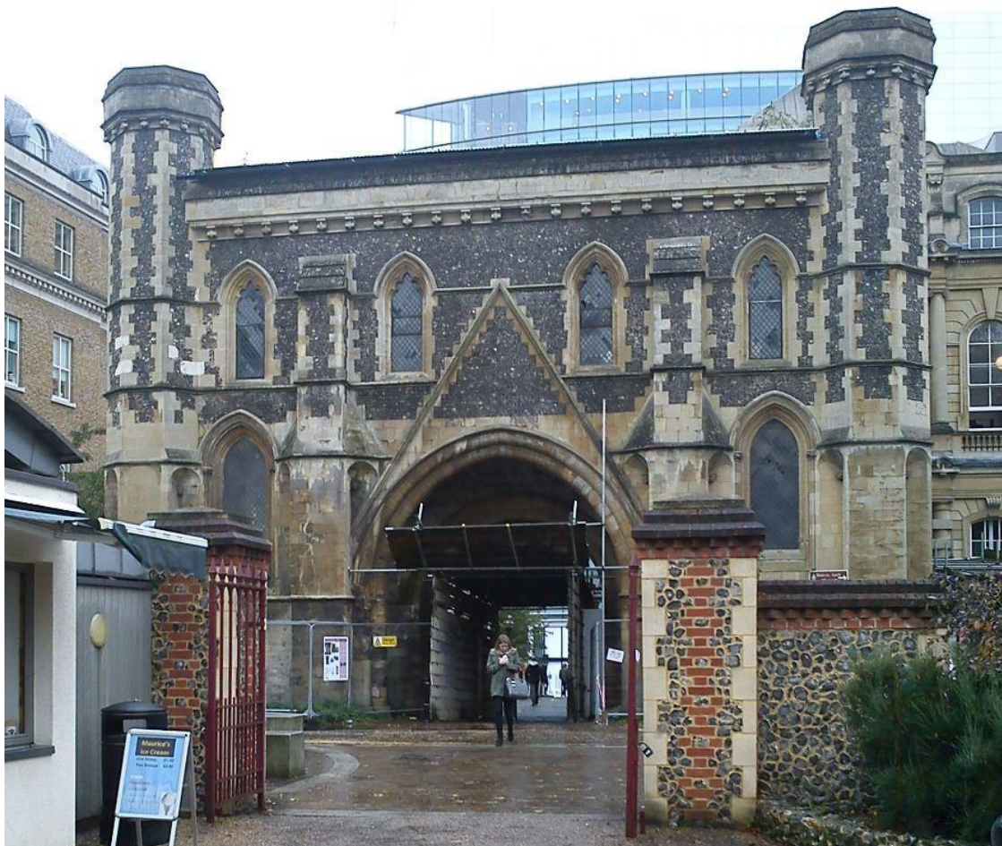
8. Photograph of the north side of the Gate in its current state with scaffolding fans, fencing and temporary roof in Place. This photograph and front cover HCC Property Services
