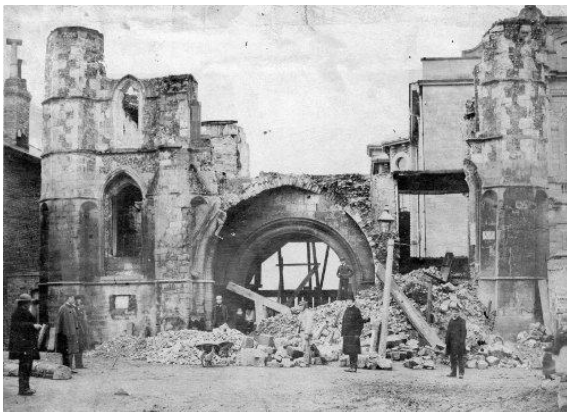
6. Partial collapse and dismantling in 1861 Reading Borough Council
