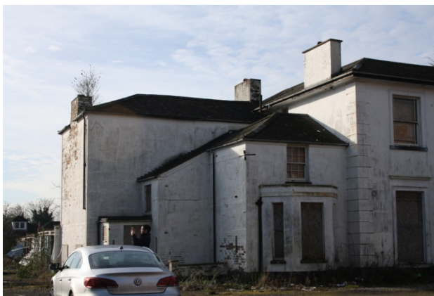
North and part of east elevations of ad-hoc arrangement of “additions” to east of main house
