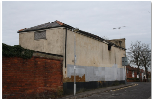
South and east elevations of the Outbuilding and part of red brick boundary wall alongside Garnet Hill
