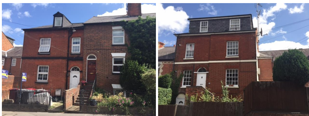
Southampton Street elevation including numbers 189 and 191 (left image) and number 187 (right image)
