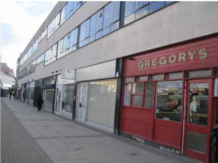
Plate 6: View eastwards along the retail parade which is now vacant.
