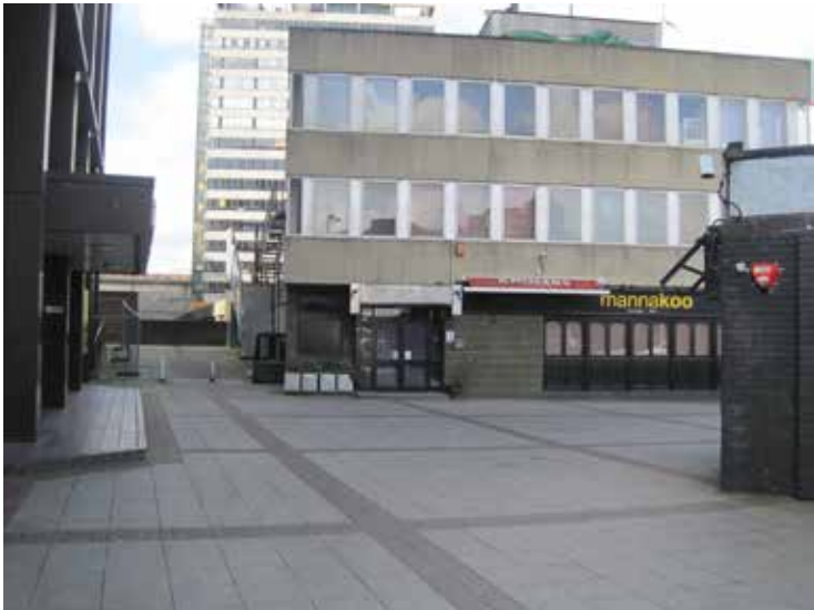
Plate 4: View westwards towards the three storey building.
