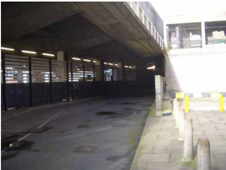
Plate 8: View northwards at the entrance to the underground car park below the Site.
