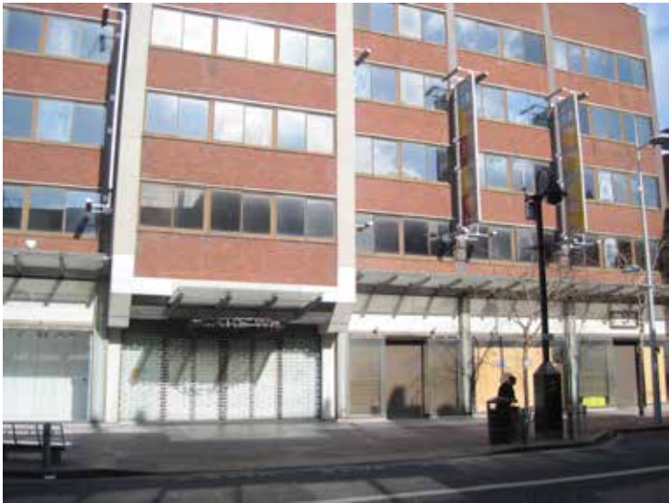
Plate 10: Friars Walk Shopping Centre fronting Friar Road.
