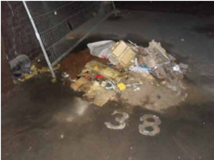
Plate 17: View of debris/rubbish in the basement carpark of Telecom House. Significant area of oil staining is visible.
