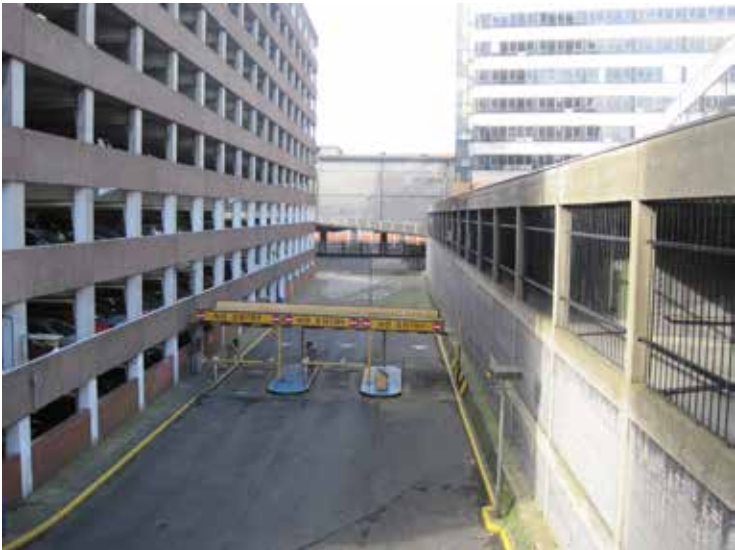
Plate 5: View westwards along the southern side of the three storey building. The brick wall encloses the underground car park. Western Tower is visible in the background
