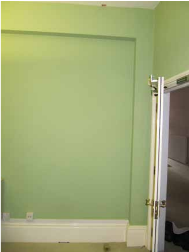
Photograph 2 - Step in wall in sever room (GF06) suggesting this wall has previously been demolished and rebuilt.
