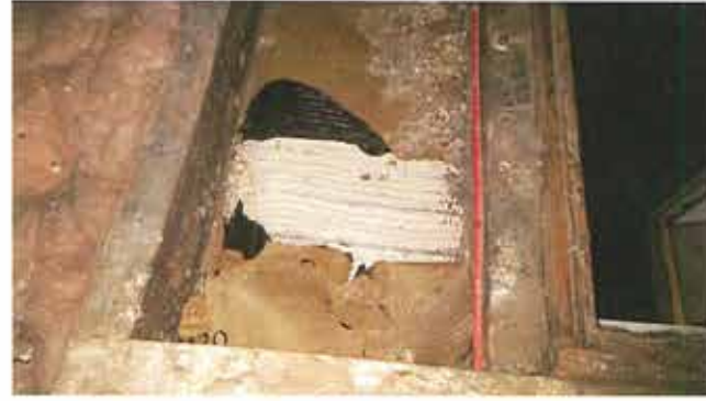
STEEL LATH CEILING
