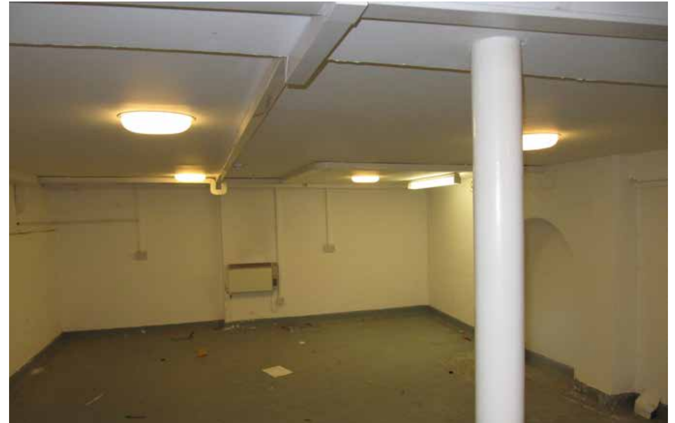
Figure 4 - The existing basement is in good condition and is ready to be used as plant and storage space.
