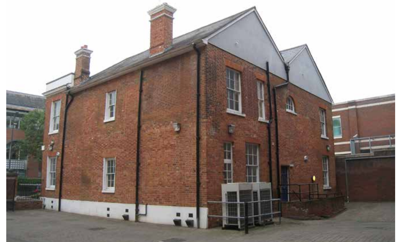
Figure 3 - Rear view of Seven Bridges House
