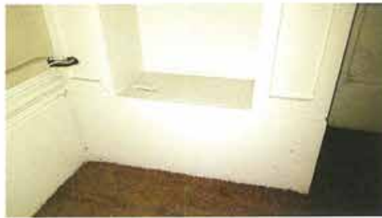
CABLES BEHIND JOINERY
