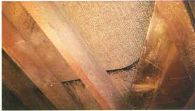
ROOFING FELT
