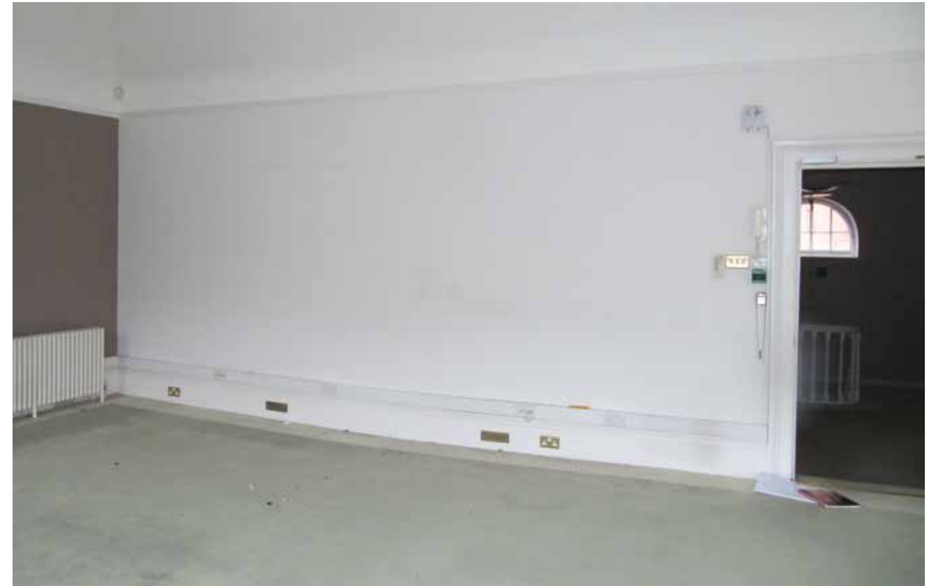
Figure 6 - The existing building's walls are peppered with services; surface mounted trunking, conduit, switches and sockets. As part of the refurbishment the majority of these services will be removed and the existing walls tidied up.
