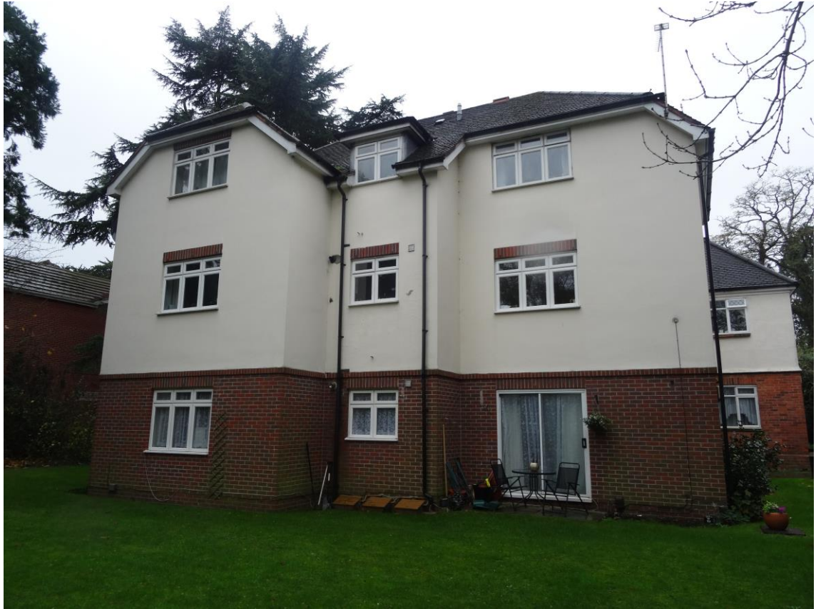
View of rear of Block 2
