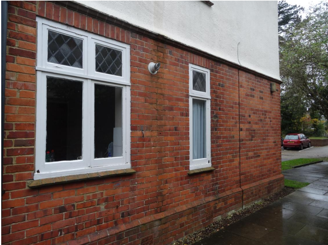
View of existing timber window of block 1
