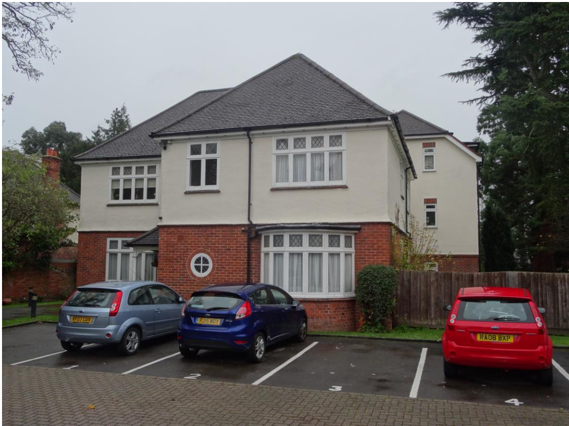
View of the front of Block 1
