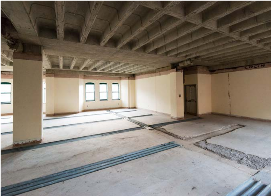
Ribbed internal concrete soffit
