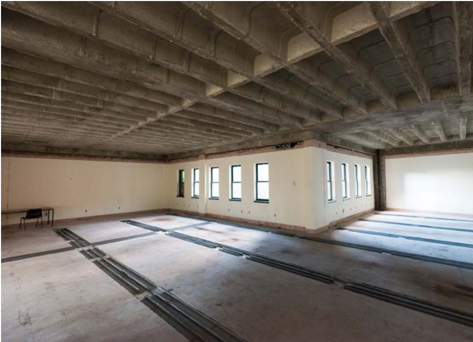
Ribbed internal concrete soffit
