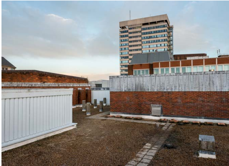
Existing Roof looking East towards Xfinity House & Great Western Tower
