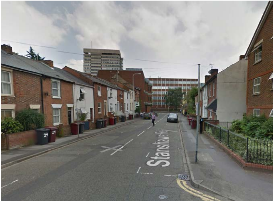
Party Wall between existing building and terraces on Stanshawe Road
