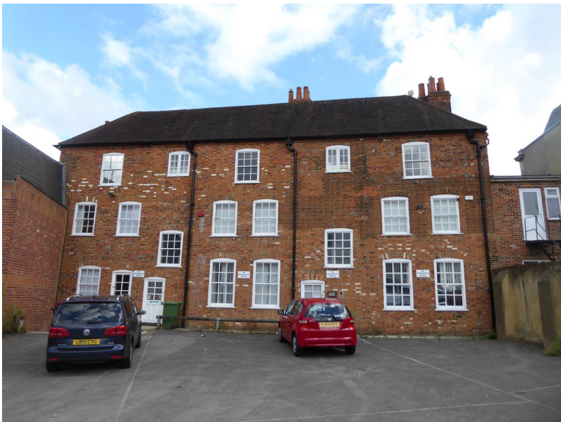
Plate 2: 54-58 London Street, rear elevation
