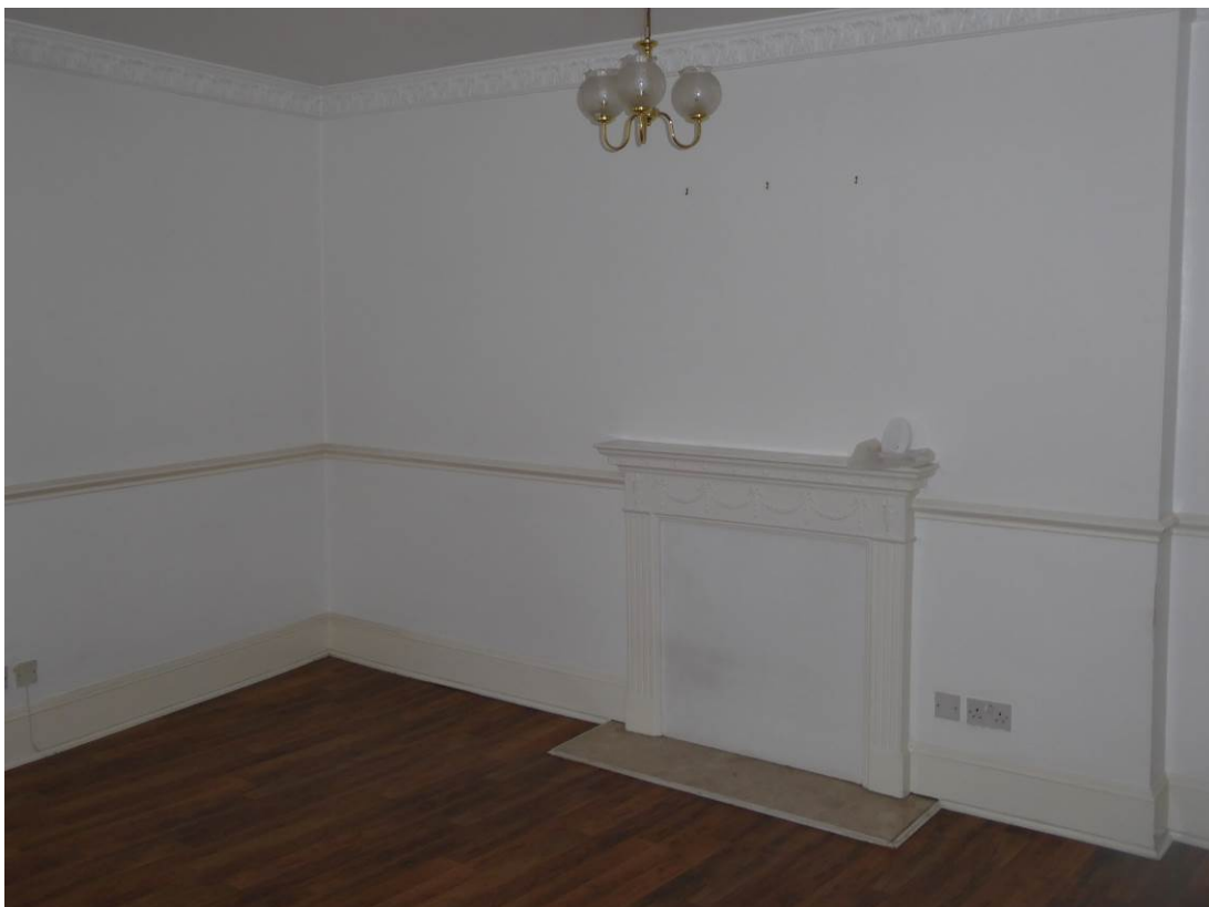
Plate 5: Ground Floor blocked modern fireplace
