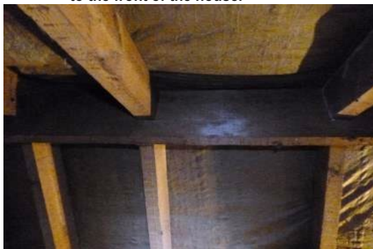
9. The hipped roof with a ridge beam which was lightly cobwebbed.
