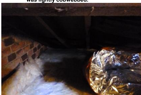
11. Fibreglass insulation extending to the eaves.
