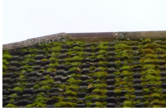
4. The ridge and hip tiles all in place and mortared fully.
