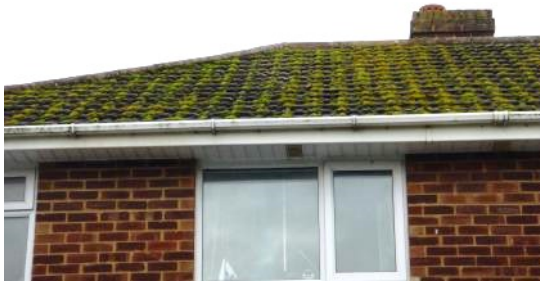
3. Interlocking roof tiles tightly fitted on the roof.
