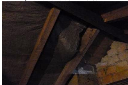
10. Paper backed felt sagging in places.
