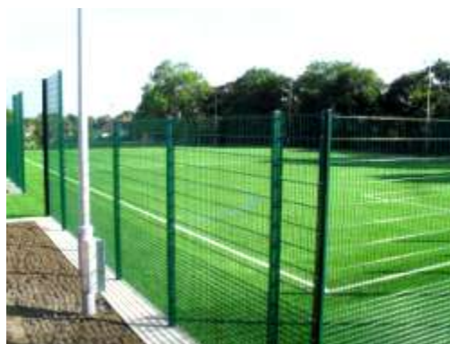
Example of ball-stop fencing
