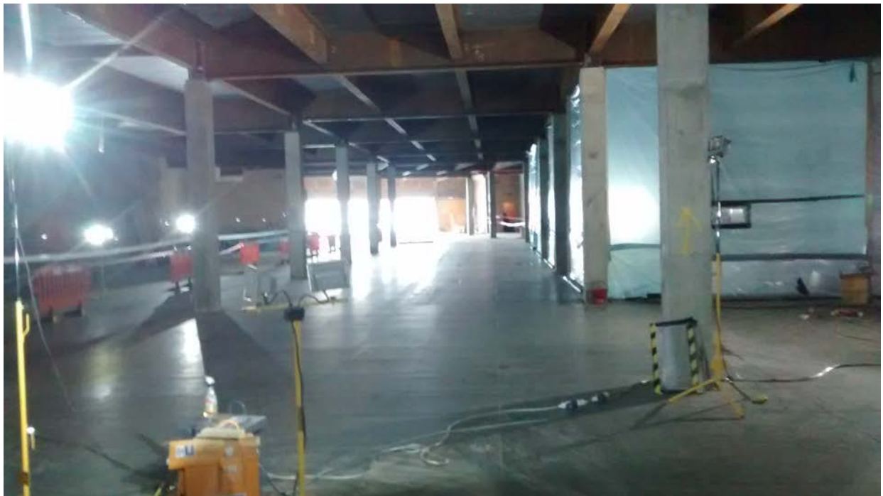
Internal view at ground floor level during the officer site visit (01/09/15)
