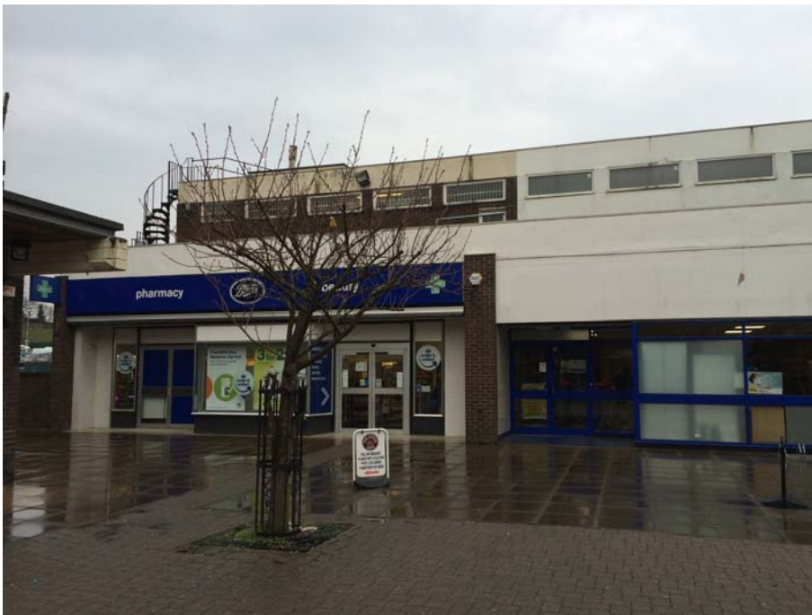
Photograph 1: Part East Elevation looking towards Boots Retail.
