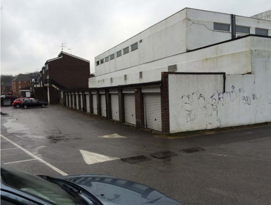
Photograph 6: Existing garages along north elevation.
