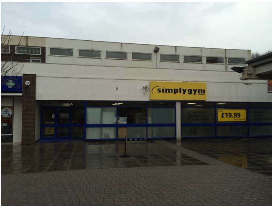
Photograph 2: Part East Elevation looking towards the Health Club adjacent to Boots Retail.
