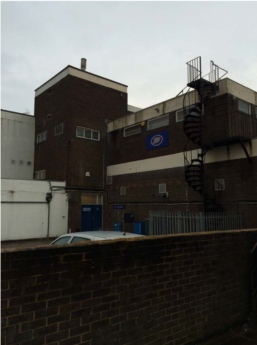
Photograph 3: Part South Elevation looking towards the rear of Boots Retail.
