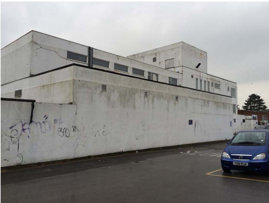
Photograph 5: West Elevation from the rear car park.
