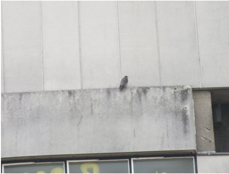
Photograph 3 -Peregrine on Western Tower – part of the open area below the roof where the birds have nested in the past can be seen on the right hand side of the picture
