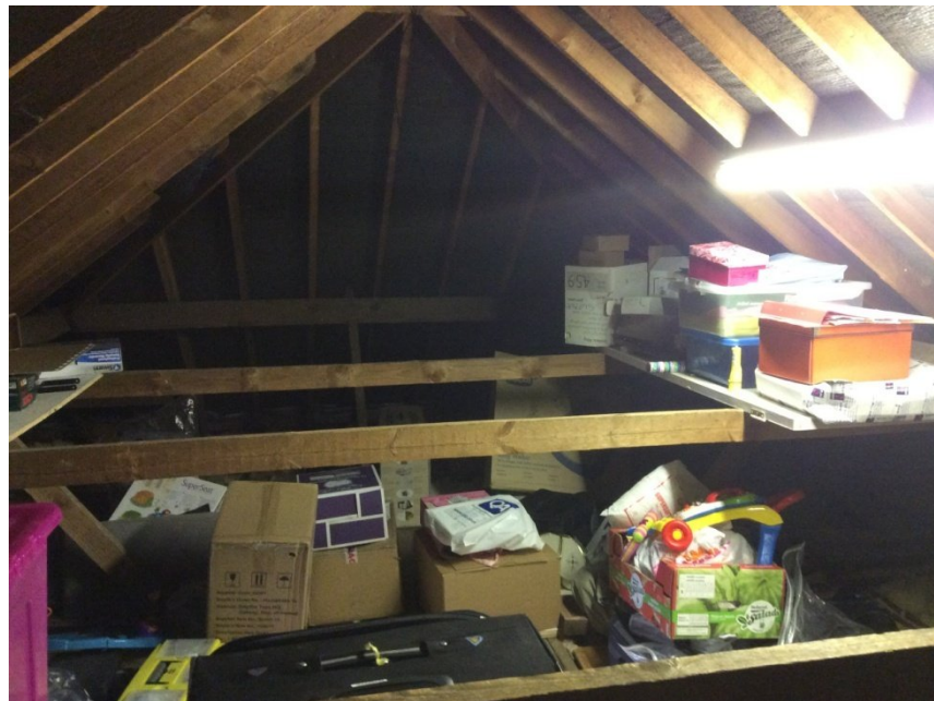
Figure 4. The larger, timber framed roof void within the northern section of the house at 60 Redlands Road.
