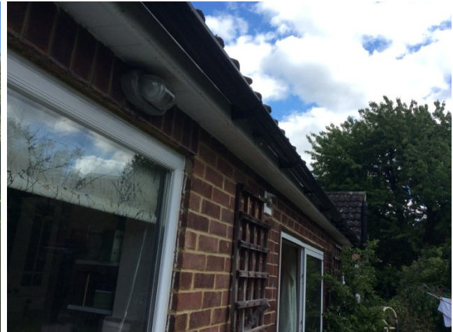
Figure 3. Well fitting, PVC soffits upon the west facing elevation of the bungalow at 60 Redlands Road.
