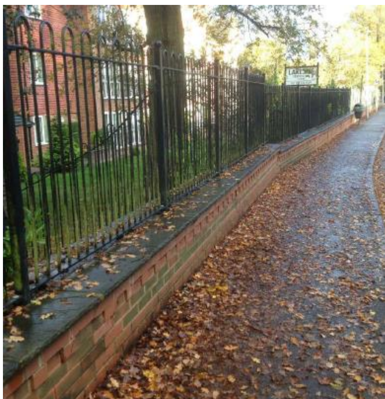
Figure 2: Image of Existing Care Home Wall to be Matched
