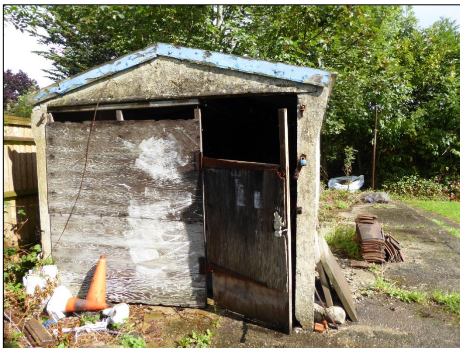
Figure 4. Garage of 26 Woods Road. 15.09.2015.
