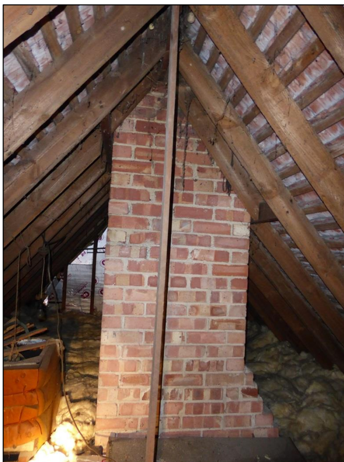
Figure 9. 26 Woods Road, roof voids, 15.09.15.
