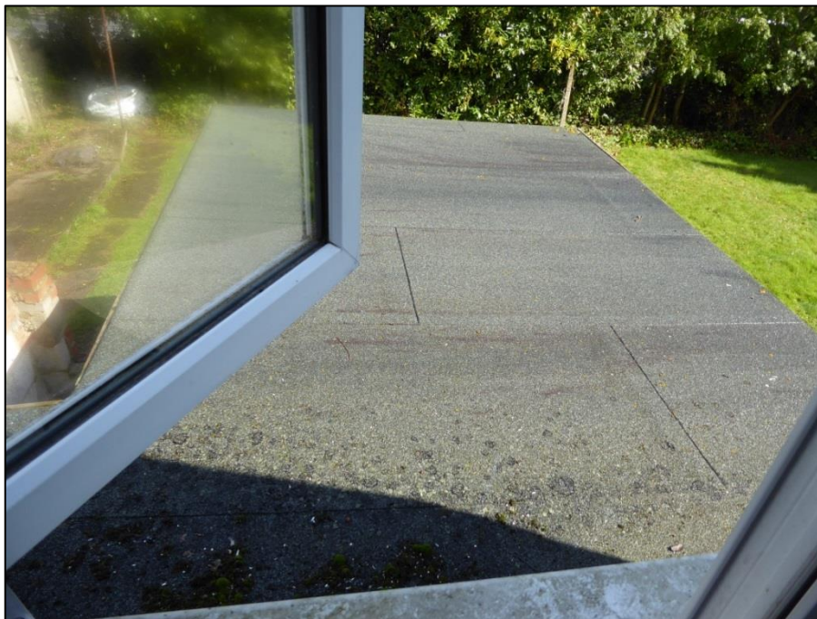
Figure 8. 26 Woods Road, rear kitchen roof, 15.09.15.
