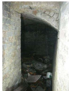
Photograph 30: Coal store viewed from B3
