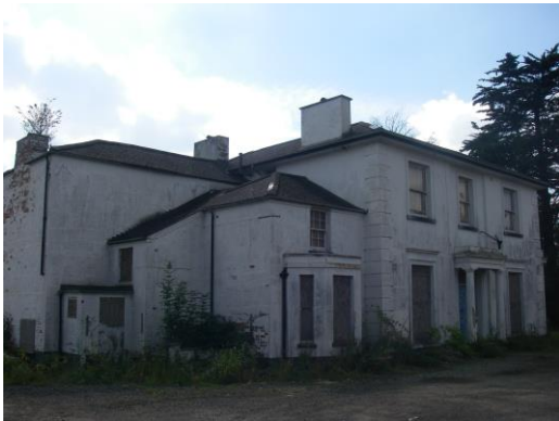
Photograph 1: Listed building viewed from Castle Crescent boundary
