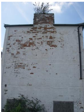
Photograph 34: Gable end of eastern addition
