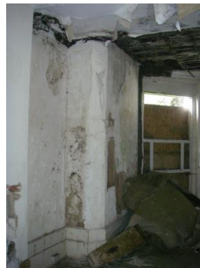
Photograph 3: Wall to bay window in G1
