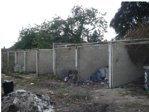
Photograph 41: Garage lock ups to rear of building
