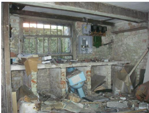
Photograph 29: Light-well window to B3
