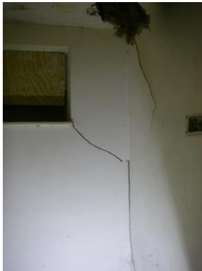
Photograph 14: Cracks to walls in corner of entrance porch in Eastern Addition
