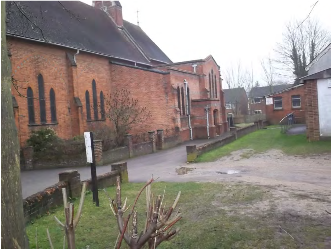
Photograph 1: Bare earth visible at current site entrance.
