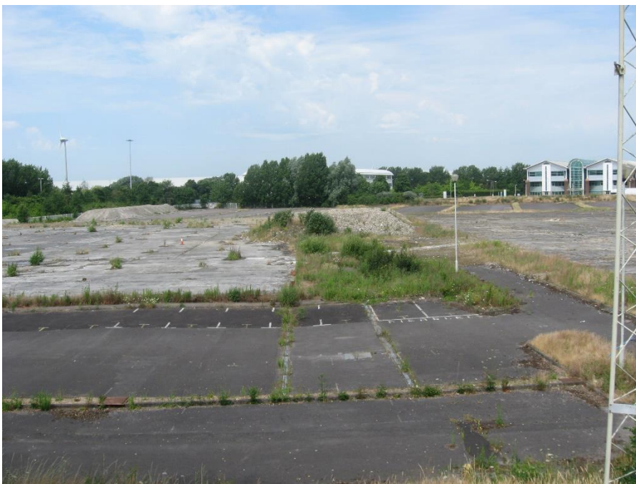
Plate 1 – The majority of the Site comprises hard standing as a result of the footprint of the former HP office buildings and associated car park areas. Sparse patches of vegetation were recorded within cracks of the hard standing.
