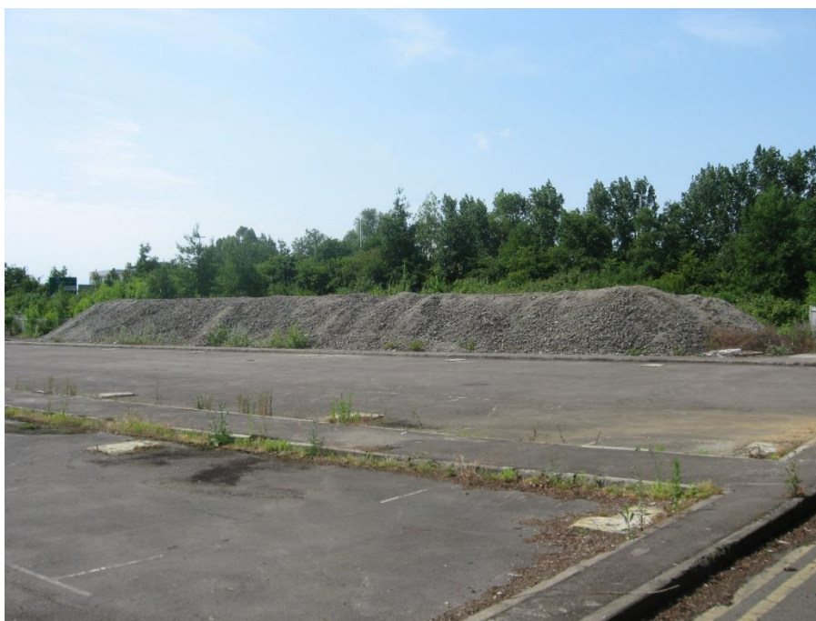
Plate 2 - Seven rubble piles, which are presumed to be the remains of the demolished HP office buildings, are present at the Site.
