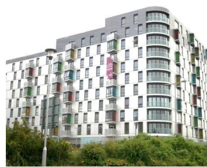
7 Chatham Street Apartments
