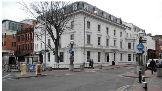
Great Western House : Grade II Listed
