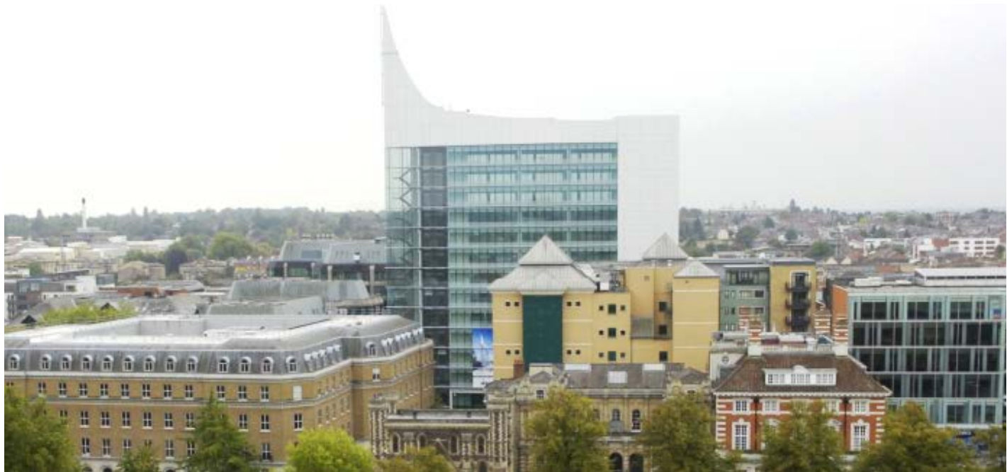
Reading Urban Landscape - Relief to and layering of building facades provides visual quality and interest when viewed from near or afar
