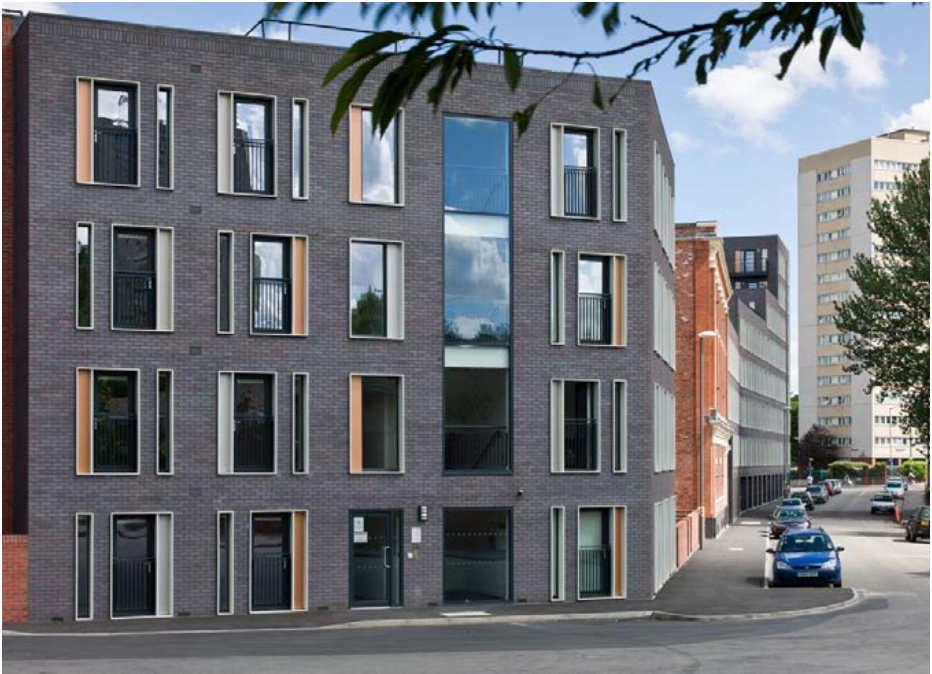
Example of brick elevation with punched brick apertures
