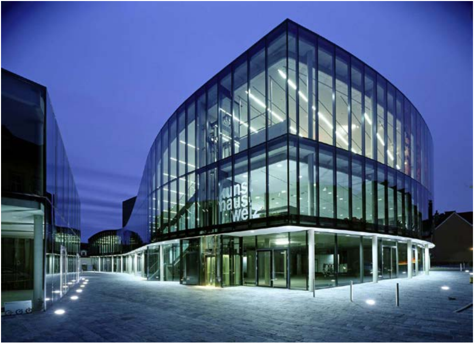
Full storey capless curtain walling - Kunst Haus, Weiz Austria
