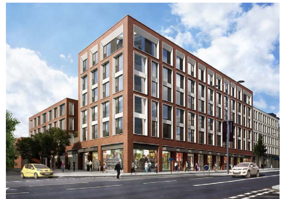
Example of brick elevation with punched brick apertures
