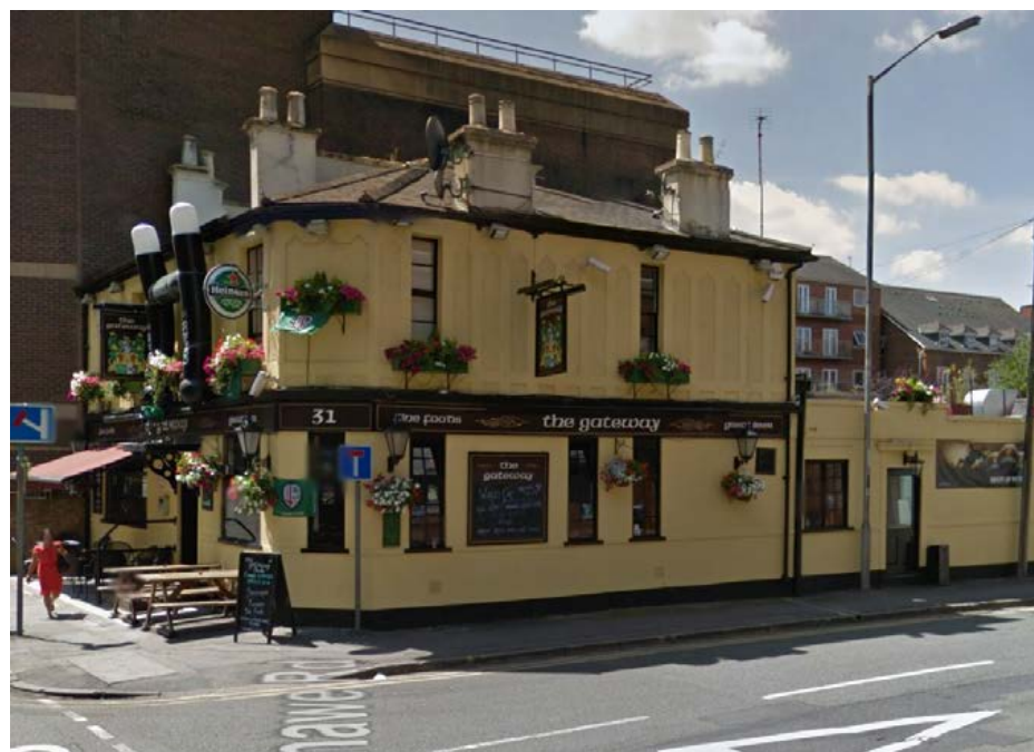
The Gateway Pub - Small upper floor windows on Stanshawe Road Elevation
