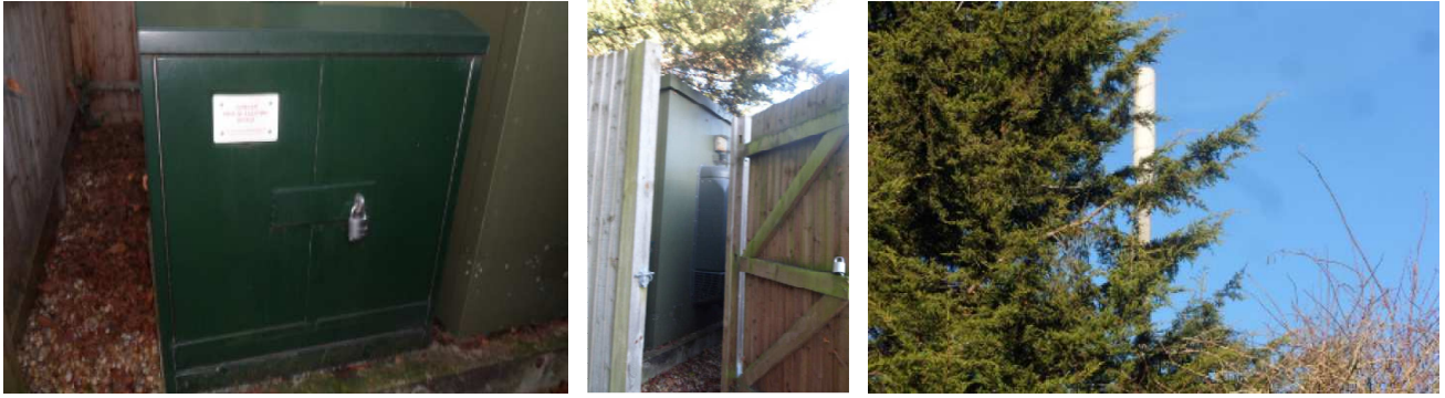
Fig. 4: Photographs showing existing meter cabinet, equipment cabin and pole
