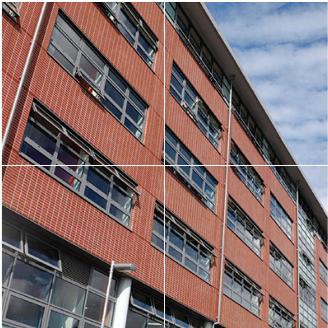
Kingspan - Mid Kent College, pre-fabricated light steel framed panels
