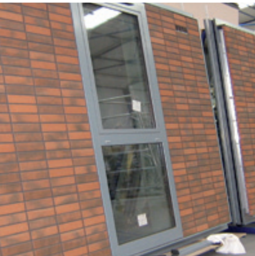
Parry Bowen Ltd - Hurst Street, Liverpool, unitised aluminium framed panels manufactured to \pm 1\text{mm} tolerance
