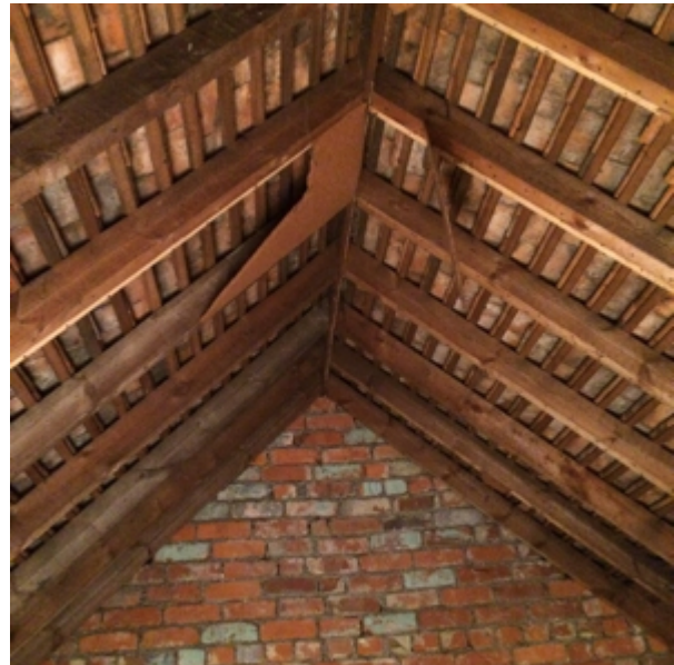
Figure 6 – Internal loft space of main roof void
