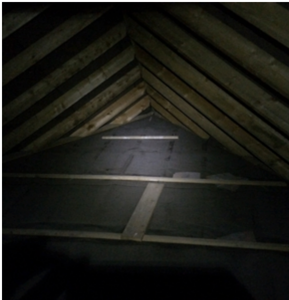
Figure 7 – Internal loft space over existing extension
