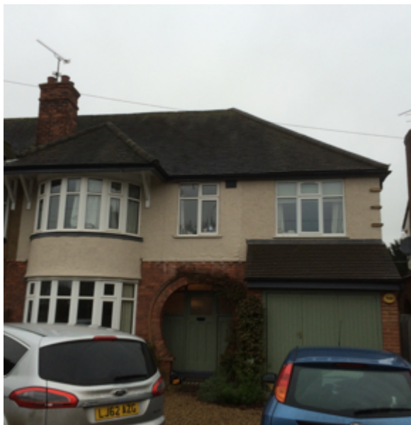
Figure 3. Front (eastern) elevation
