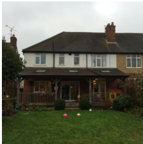
Figure 4. Rear (western) elevation
