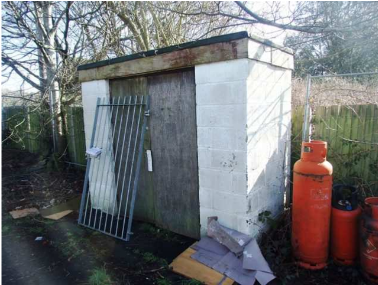
Photograph 9: The utility building.
