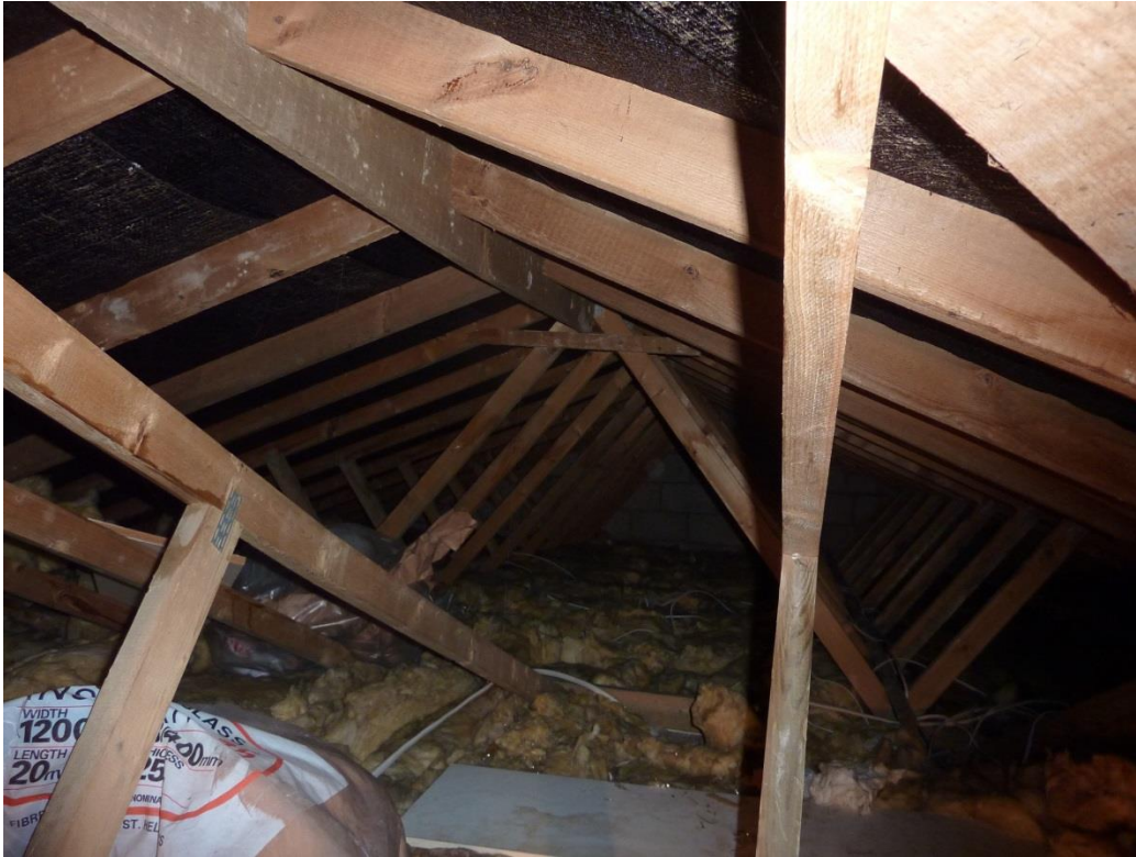
West section of roof void
