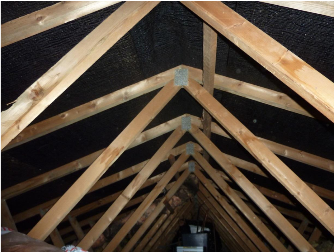
View of roof void from north gable.
