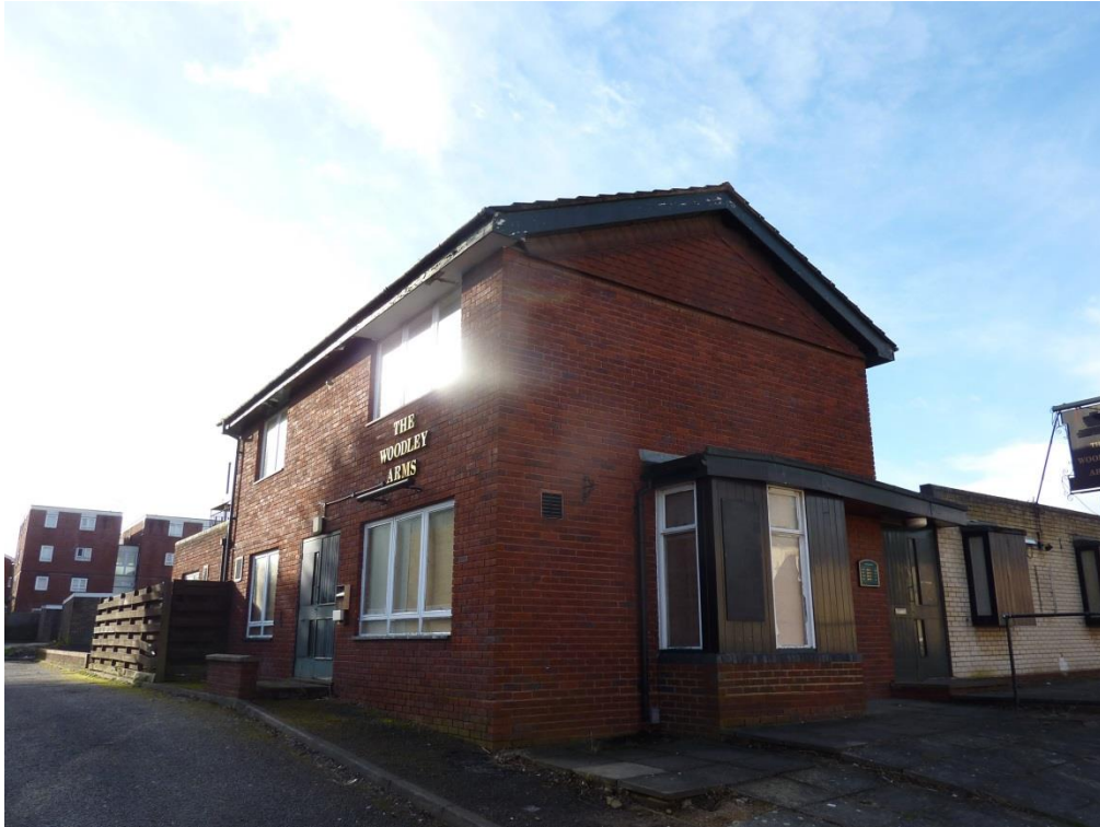
North-east view of the property showing hanging tiles
