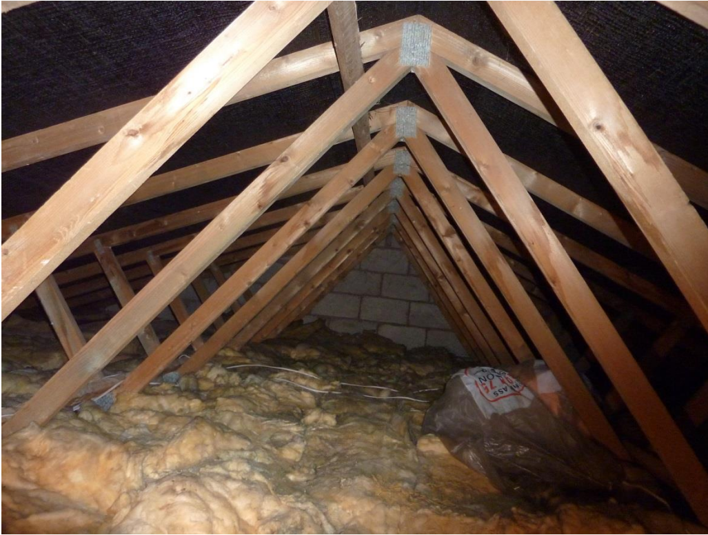
North gable end of roof void
