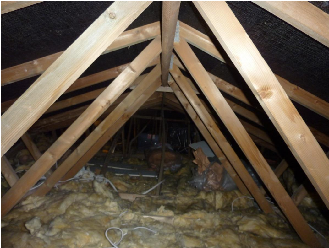
View of void from west gable wall
