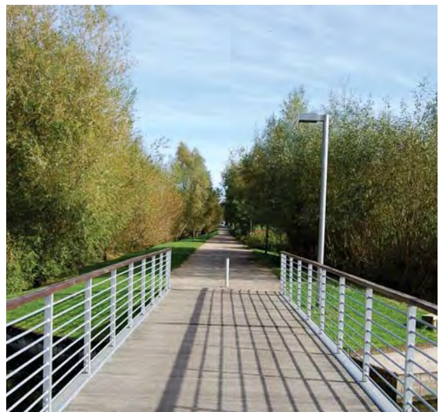
View along willow walk following construction
