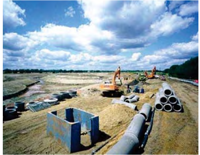
View to 100 Longwater from entrance before lake filling
