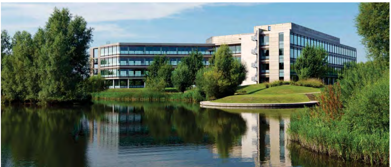
View towards 350 Longwater Avenue
