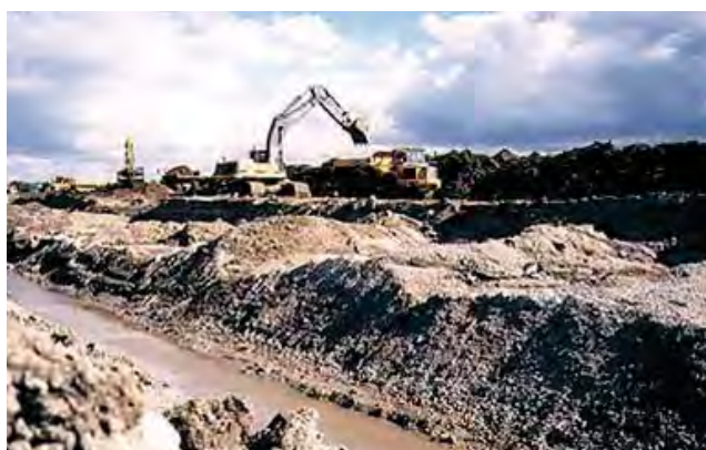
The initial works to form Longwater
