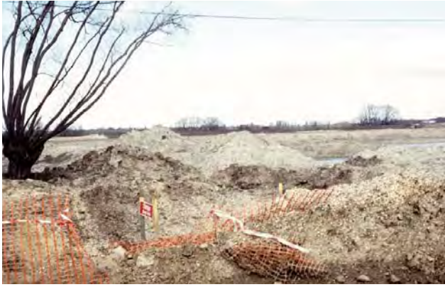
Retained willows in midst of development platform construction
