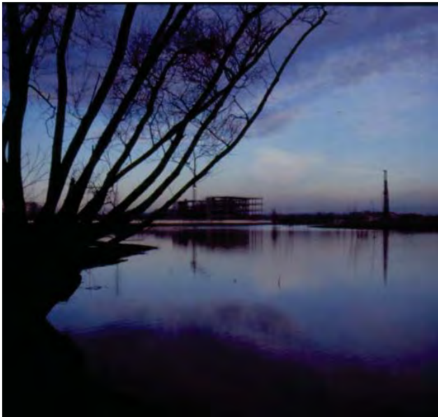
Flooding had to be anticipated during construction
