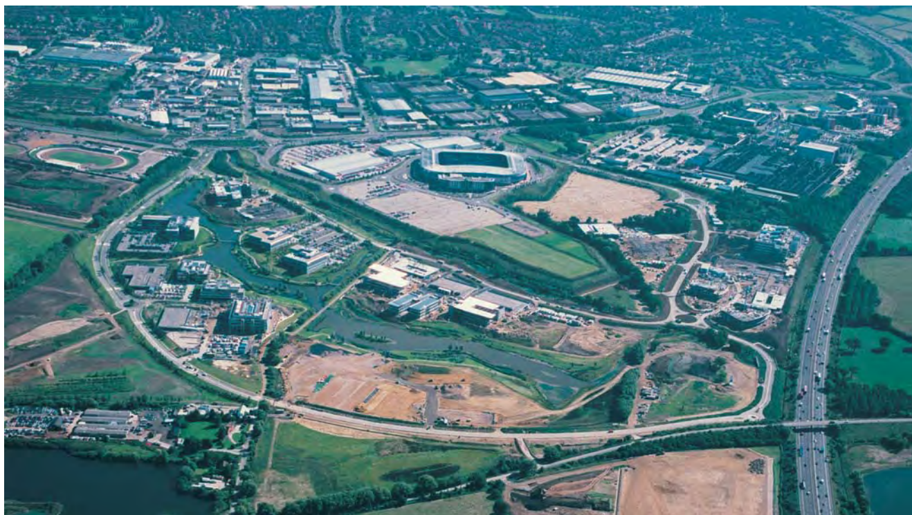
Longwater maturing in the centre of the site
