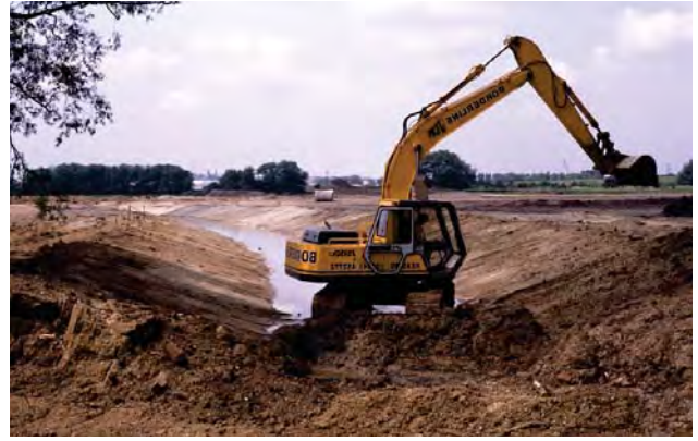
Initial formation of Longwater to allow flood waters to pass through site
