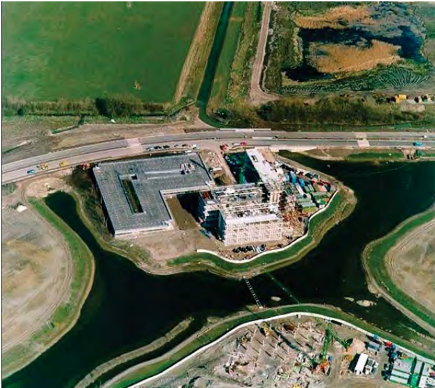
100 Longwater in course of construction
