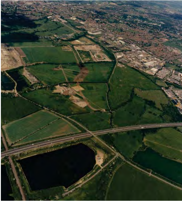
The Green Park site viewed from the south during investigative works.
