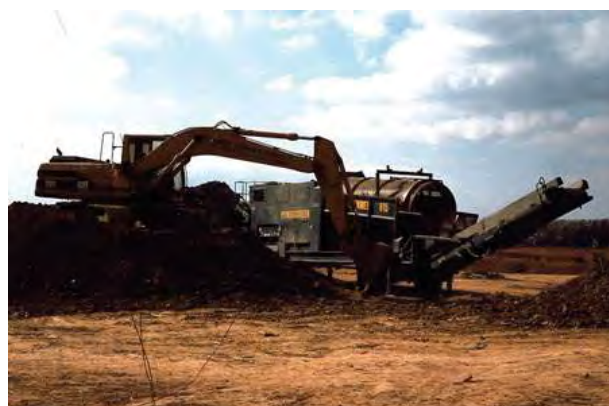
Soil preparation mixing BioGran with site soil
