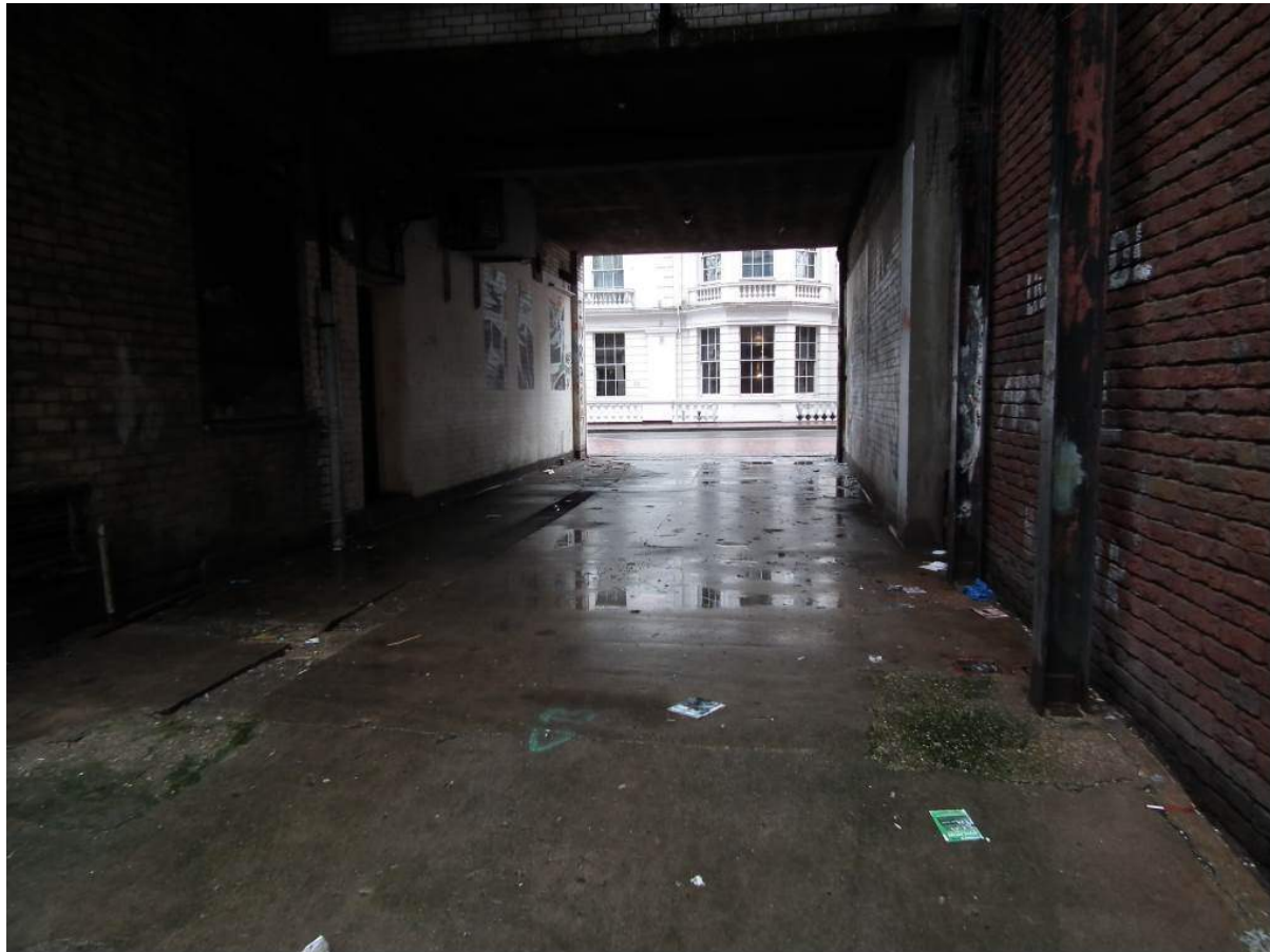
PLATE 1 –WS101 AND WS102 LOCATED IN UNDERCROFT AREA OF STATION ROAD (FACING STATION ROAD - 27/11/2014)
