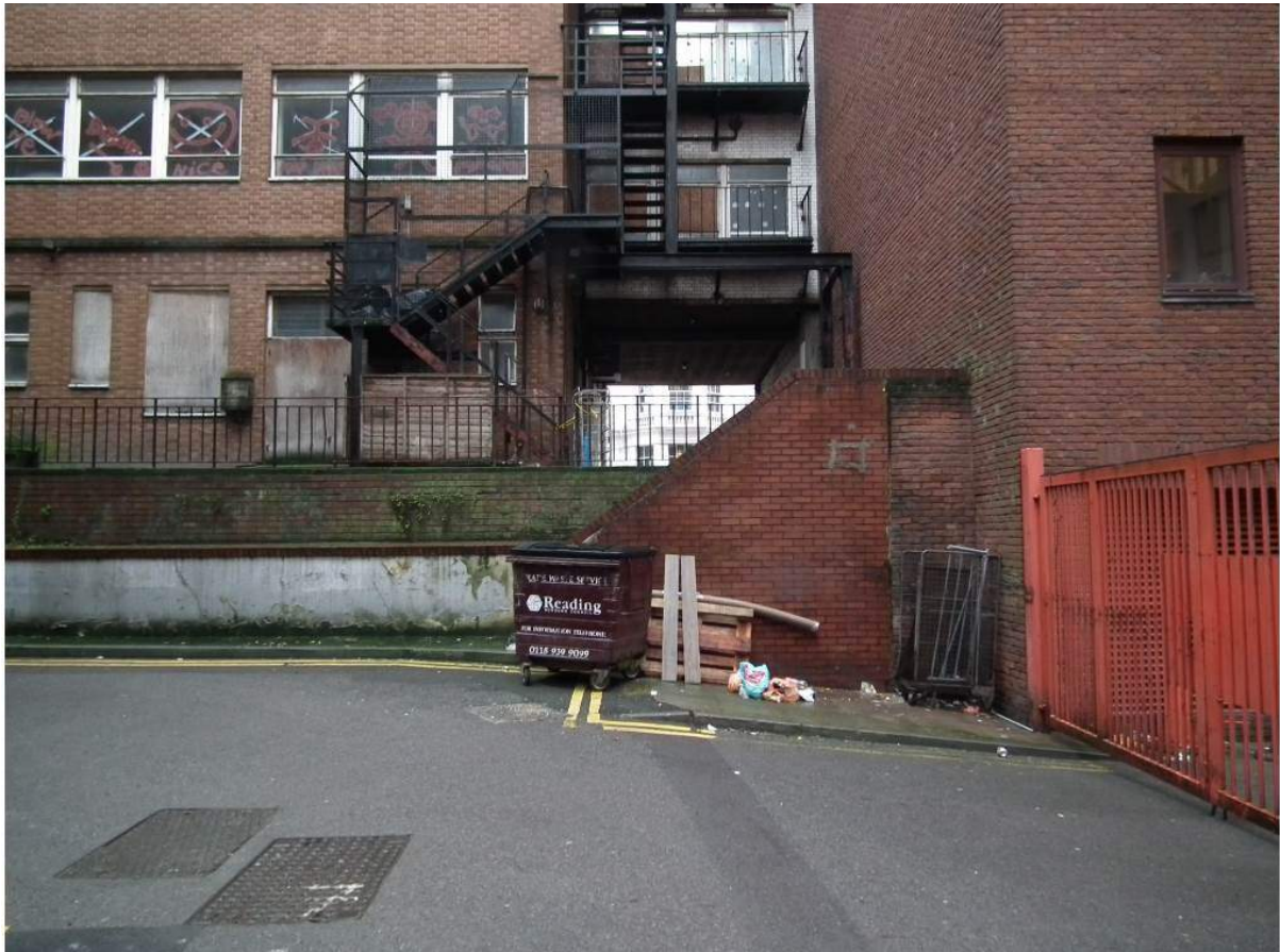
PLATE 4 – REAR OF 29-35 STATION ROAD (FACING EAST – 27/11/2014)
