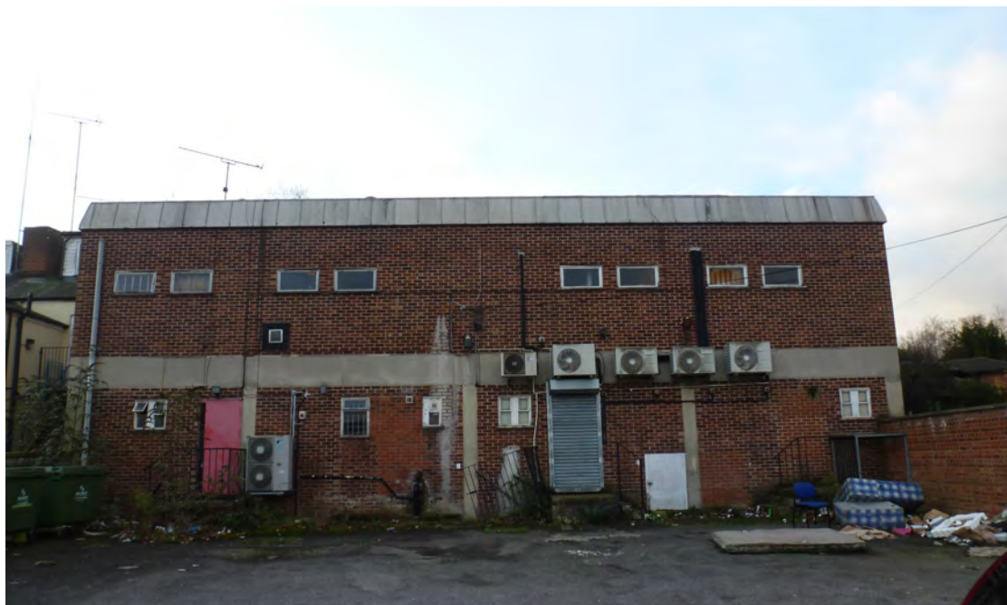
Fig.5: Existing view of the north elevation and car park at 750 and 752 Oxford Road
